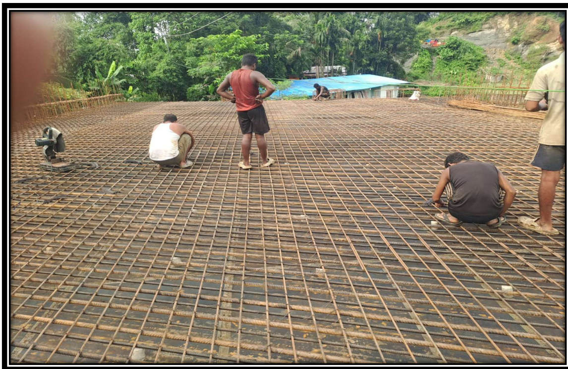
2. Reinforcement work at Ch.4+212 (LVUP)
