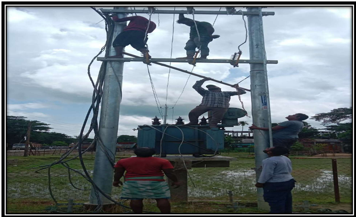
6. Utility shifting work at Ch. 13+380
