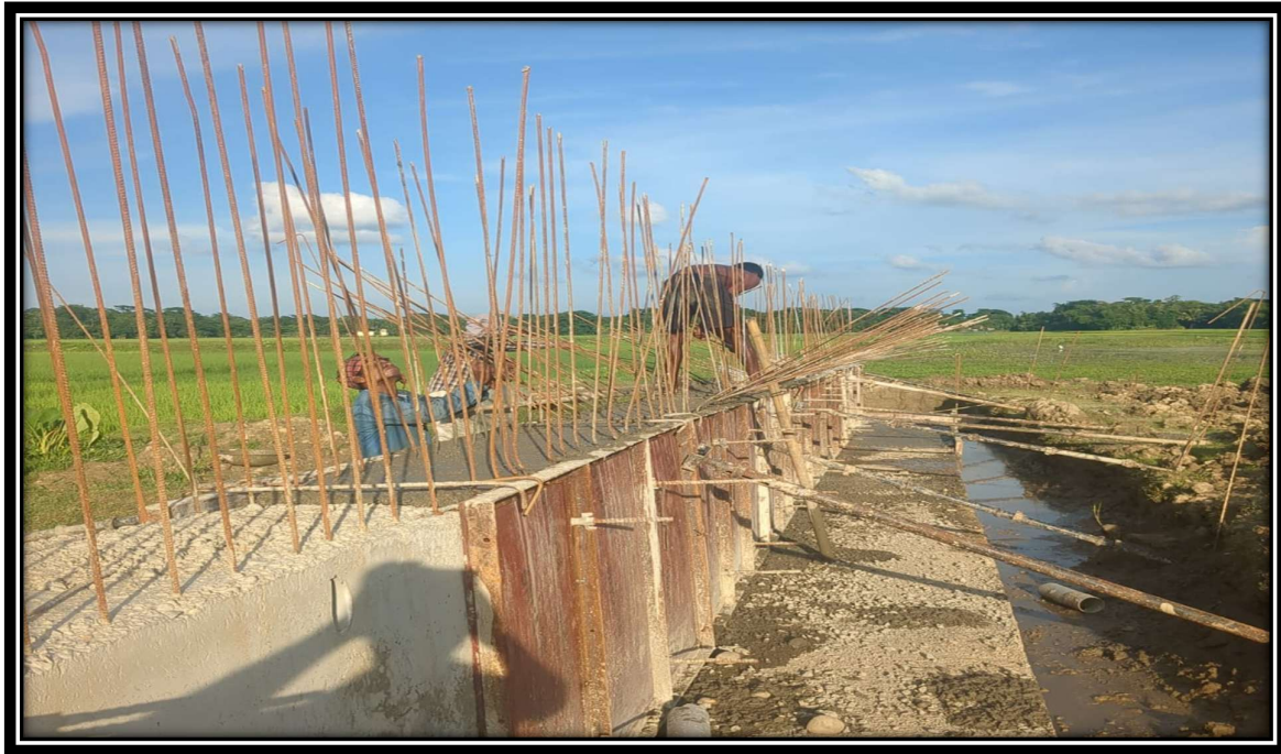
1. Concrete pouring work for Toe wall Ch. 10+050
