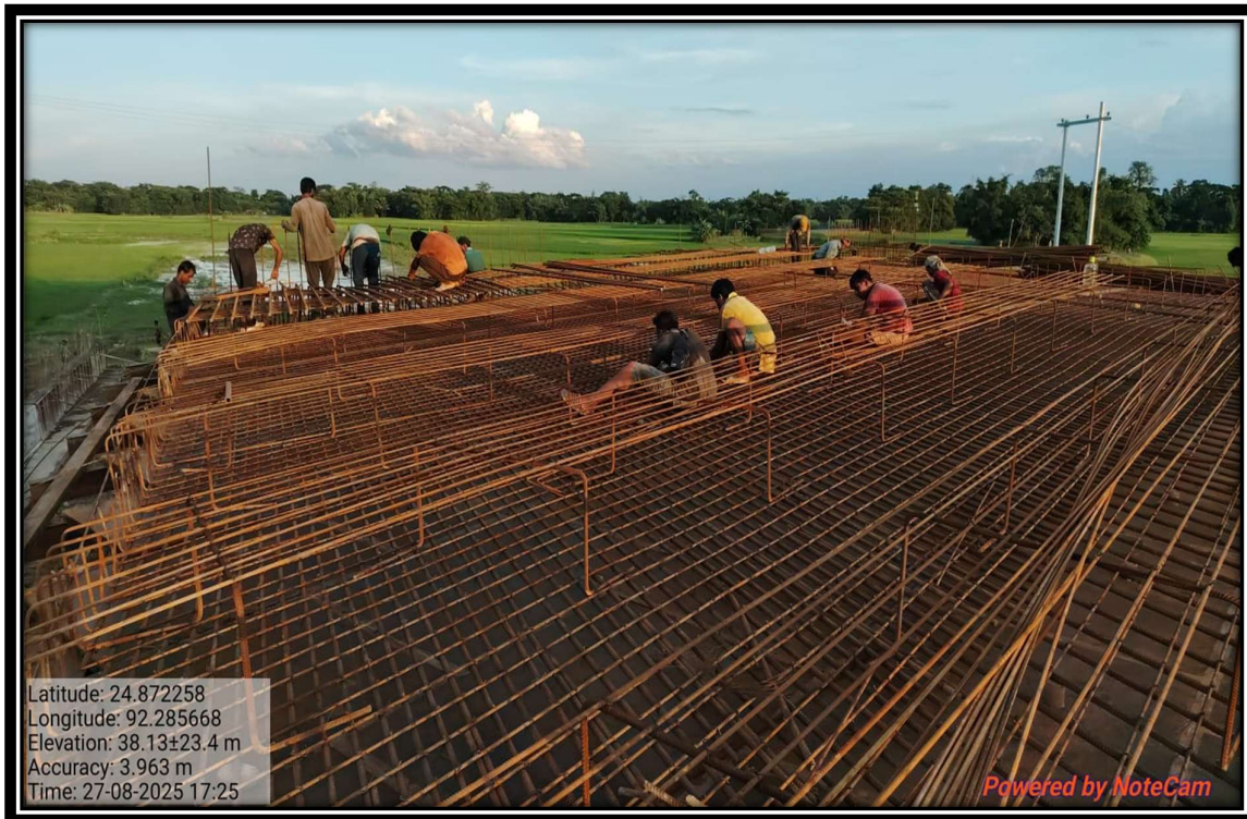
5.Reinforcement work at Ch.10+098 (LVUP)
