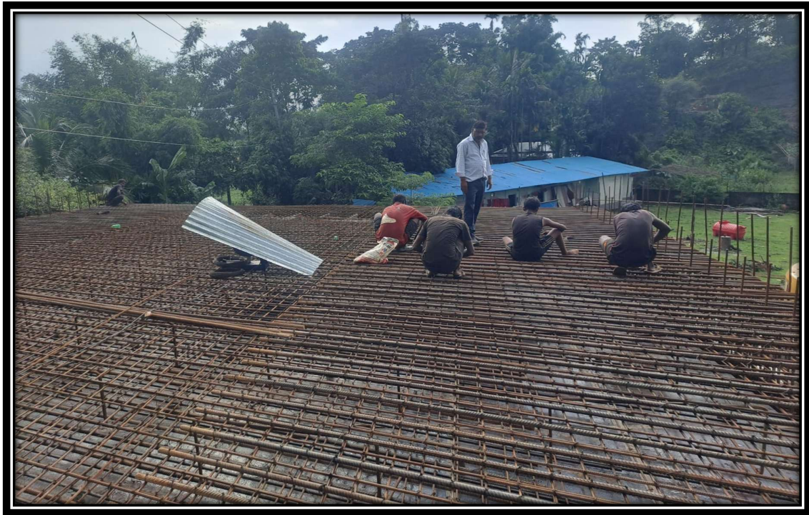
3. Reinforcement work at Ch.4+212 (LVUP)
