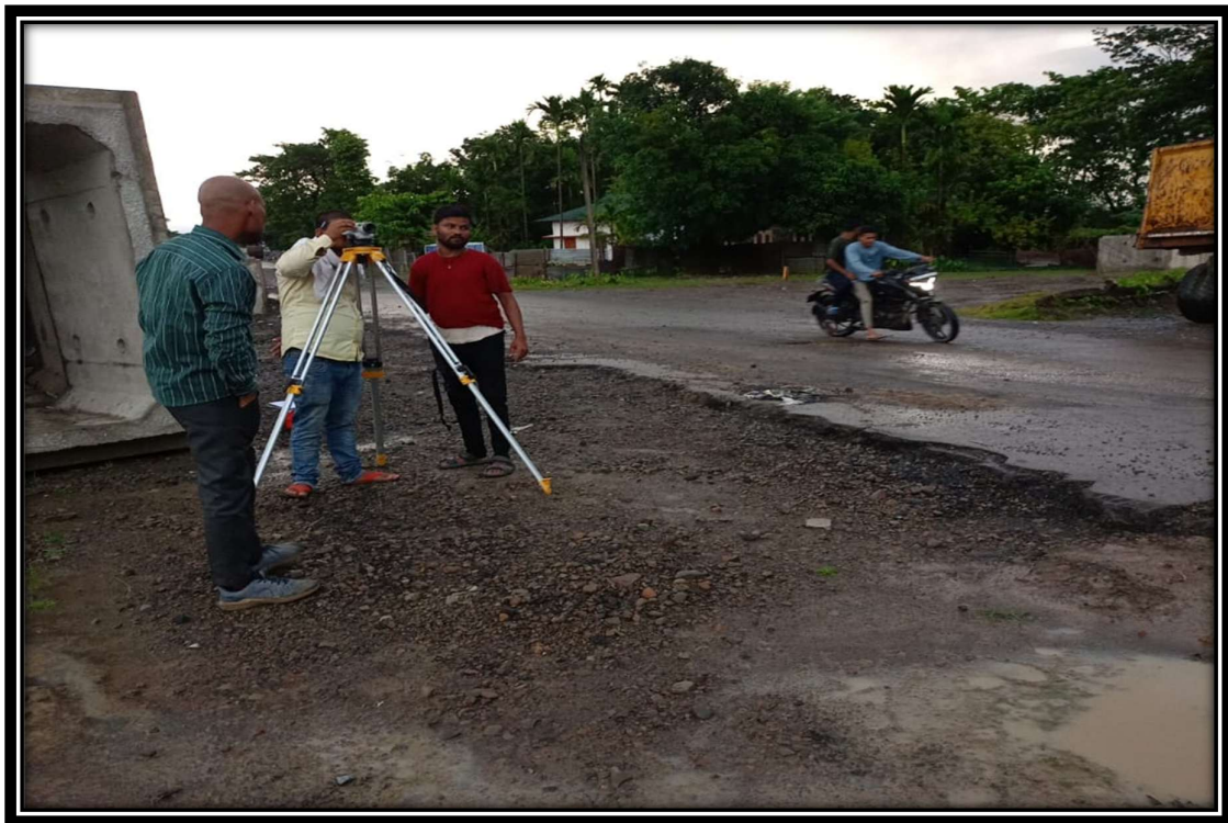
4. Level Checking work for SG top at Ch.- 12+900 to 13+200
