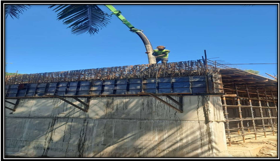
1. Concrete work at Ch.12+310 (LVUP)
