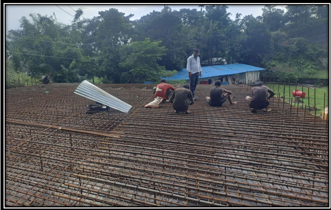
3. Reinforcement work at Ch.4+212 (LVUP)
