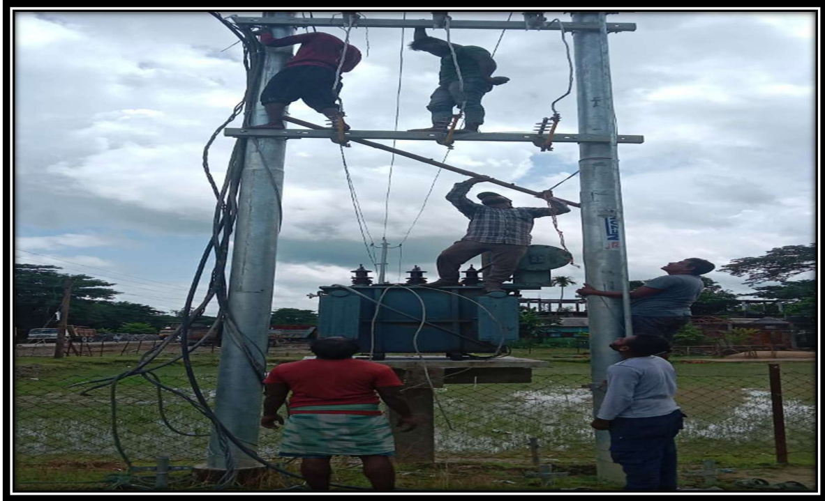
6. Utility shifting work at Ch. 13+380
