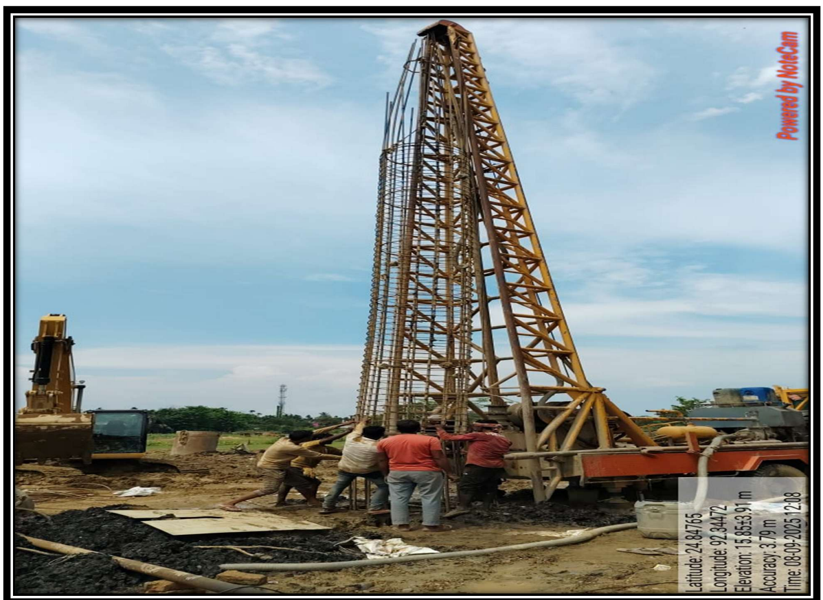
6. A2 Pile No. 03 Cage Lowering work at Ch. 2+893
