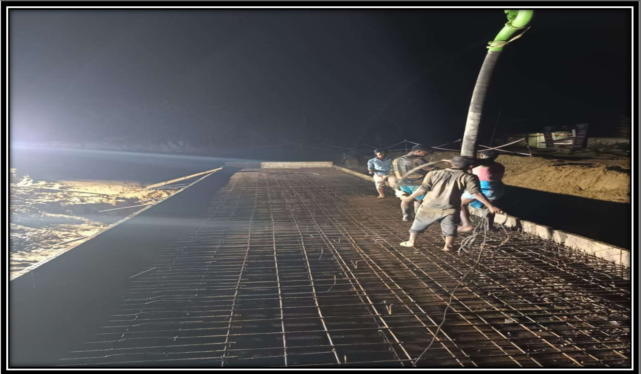
Concrete Pouring works in progress at Ch.- 92+862
