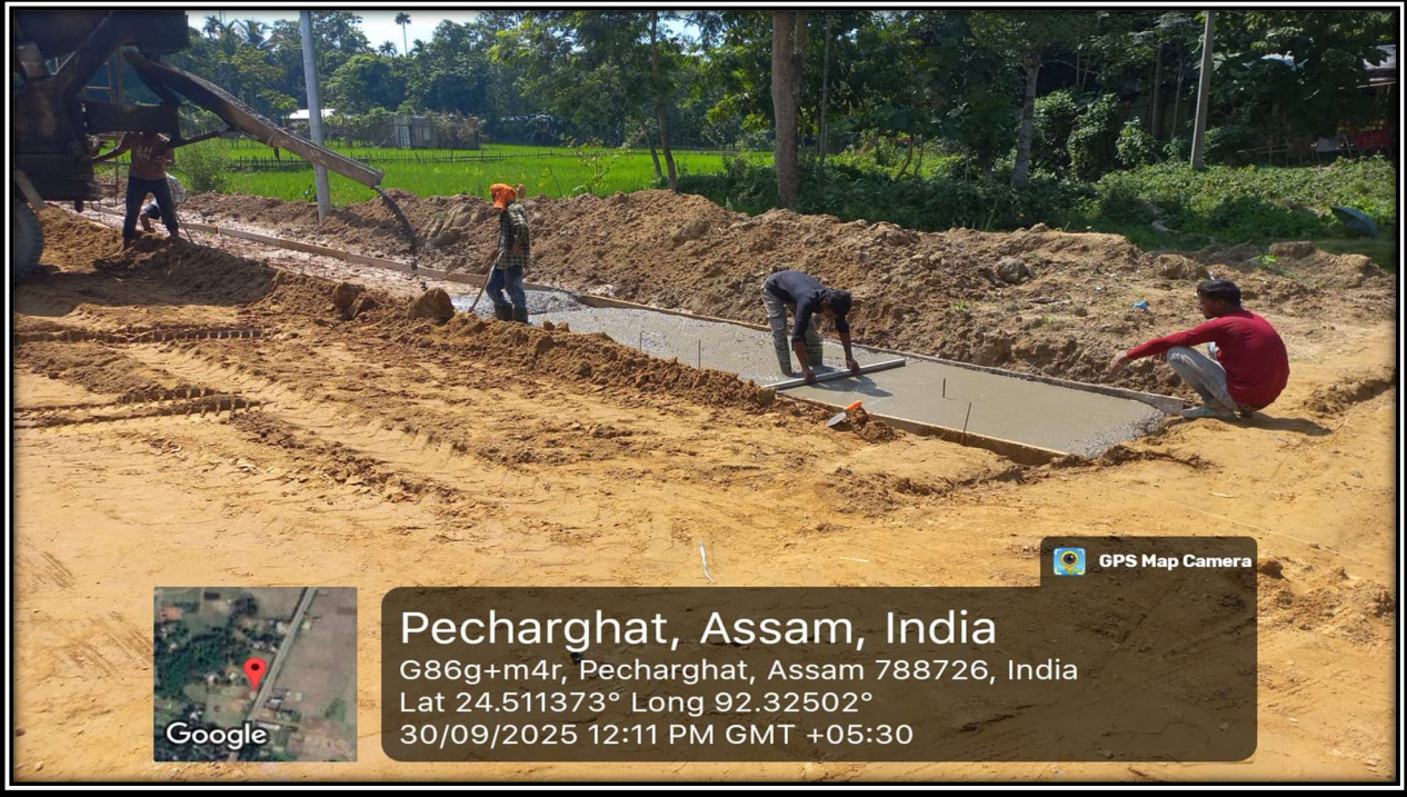
RCC Drain PCC Work in Progress at Ch.- 94+060 to 94+100 RHS
