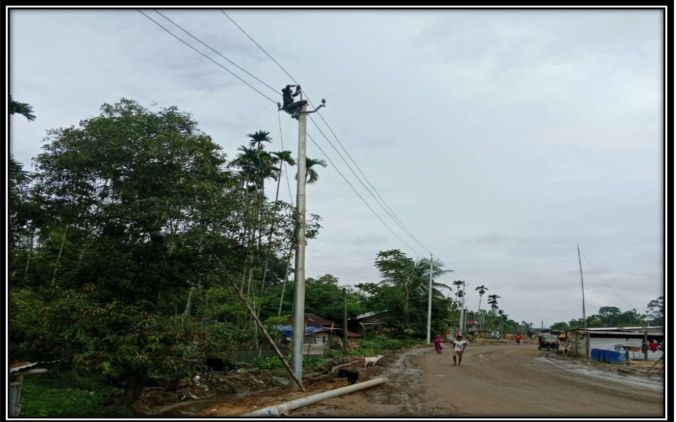
Electricity H/T line Conductor sagging work in progress at Ch.- 94+625
