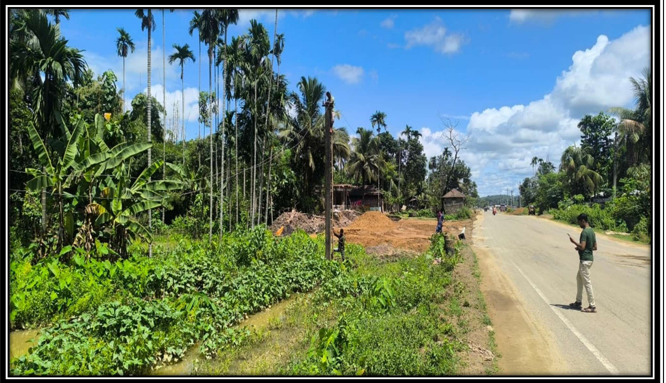
Electricity L/T line removing work in progress at Ch.- 94+450
