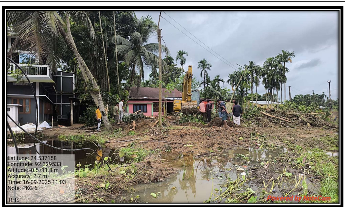
C&G work in Progress at Ch.- 91+200 RHS
