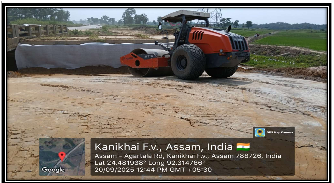
MNB Geo composite fixing & back filling & rolling work in progress at Ch.- 97+680 A2 Side
