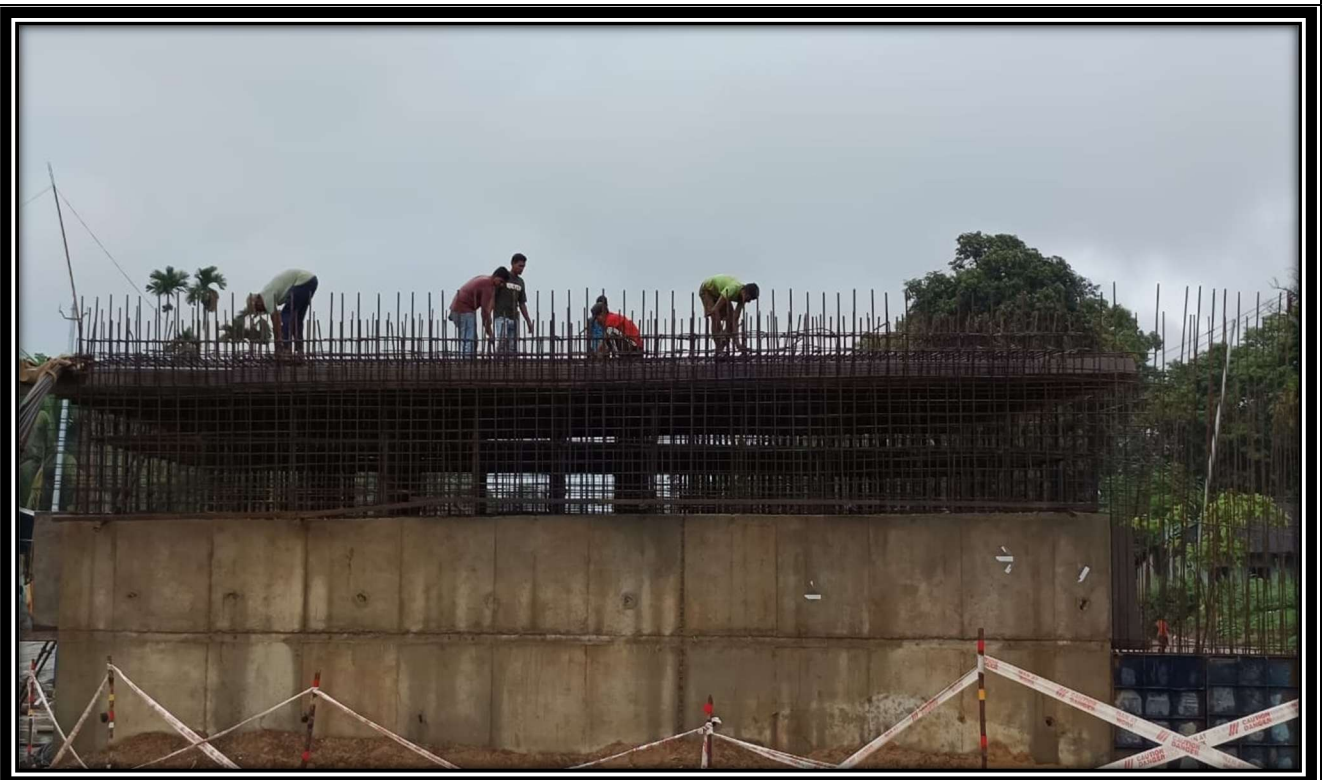
Reinforcement Work in progress at Ch.- 94+625 RHS
