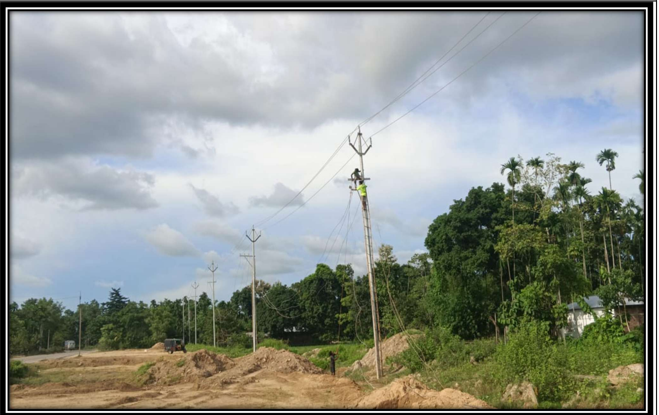
Electricity H/T line Conductor sagging work in progress at Ch.- 92+150
