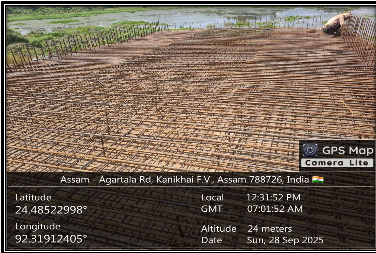
MNB Top Slab Reinforcement fixing work in progress at Ch.- 97+100 RHS
