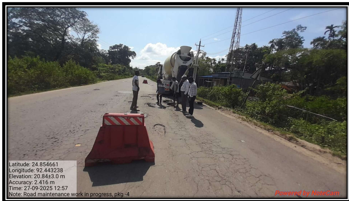
Existing Road Maintenance Work
