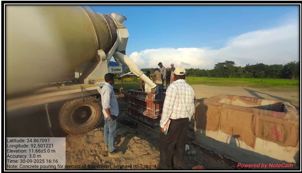
Precast Box Segment Concrete Work
