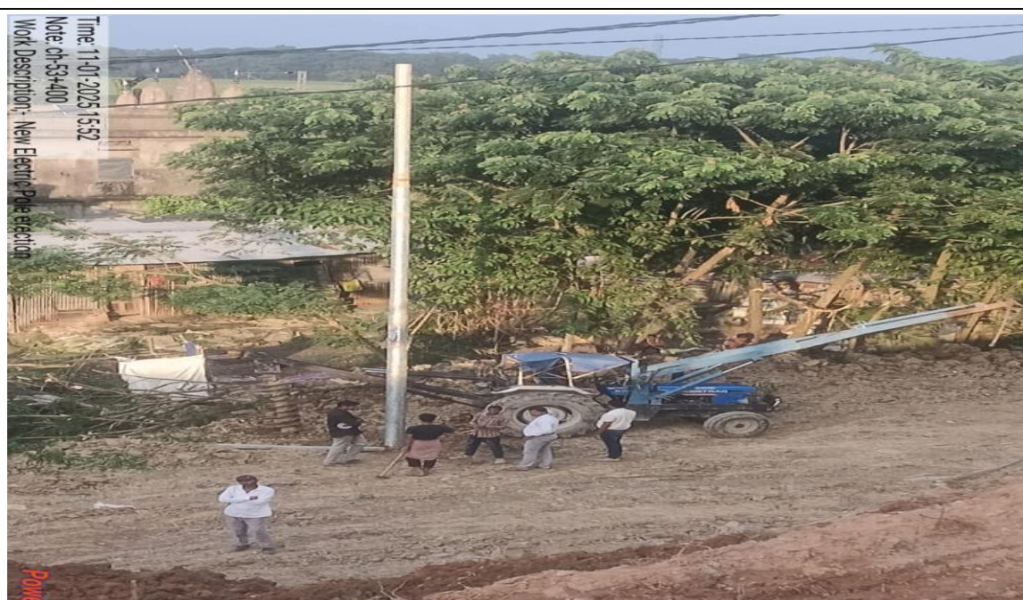
Utility Shifting in Progress at 53+300 To 54+000 BHS
