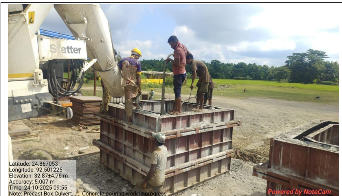
Pre Cast Box Culvert Segment at 00+300
