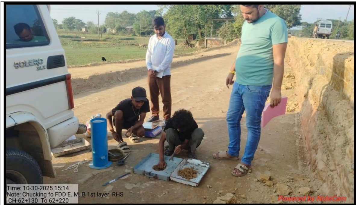
FDD Checking of Emb:- 1 st Layer
