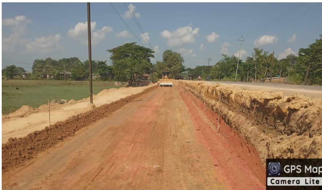
Emb Layer in progress at 62+710 to 62+800 RHS
