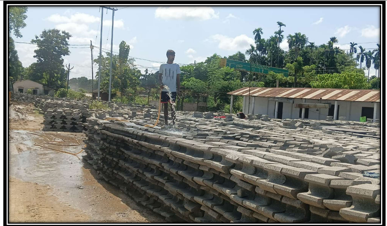
RE Block curing work in progress at Ch.- 95+100
