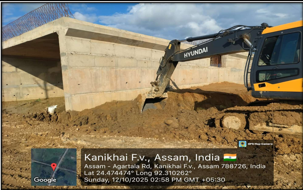
Excavation work for Retaining wall at chainage-98+587
