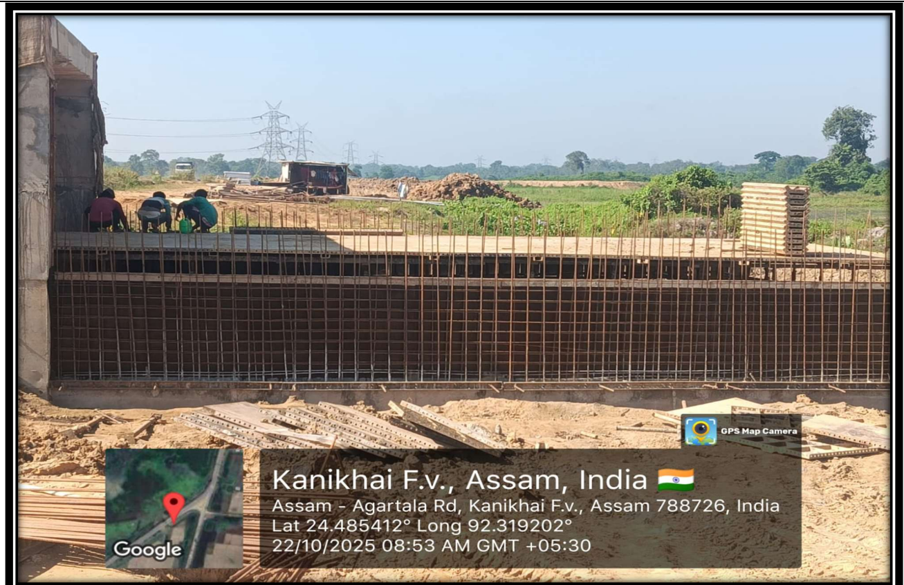
Reinforcement work at chainage-97+102 MNB (Sr.Road)
