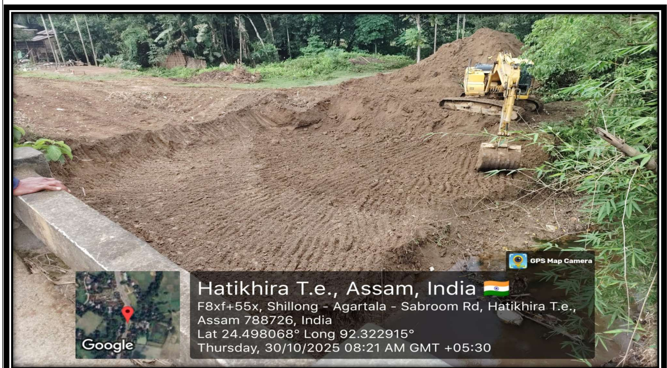
Excavation work at chainage- 95+595 (for MNB foundation)
