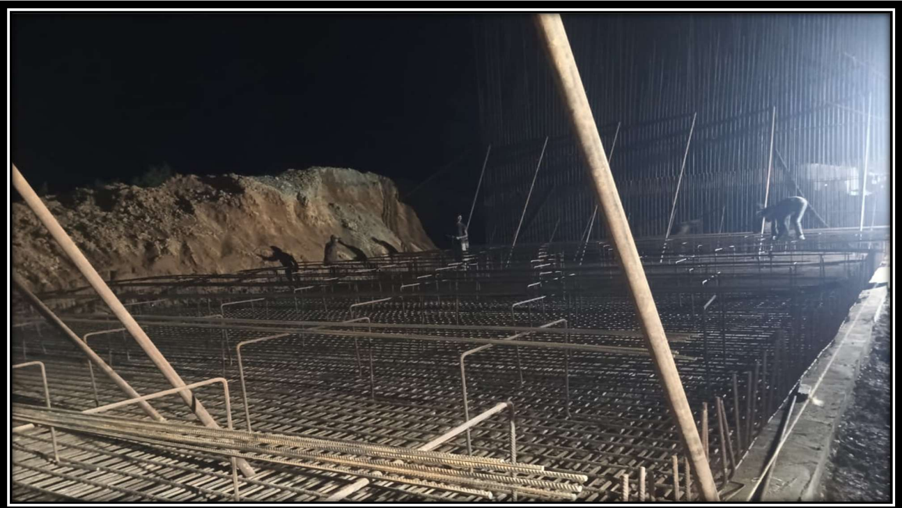
Reinforcement Placing work at 97+000 VUP
