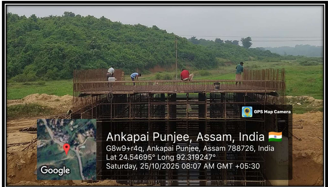
Reinforcement work for slab at chainage 89+543(Sr. Road)
