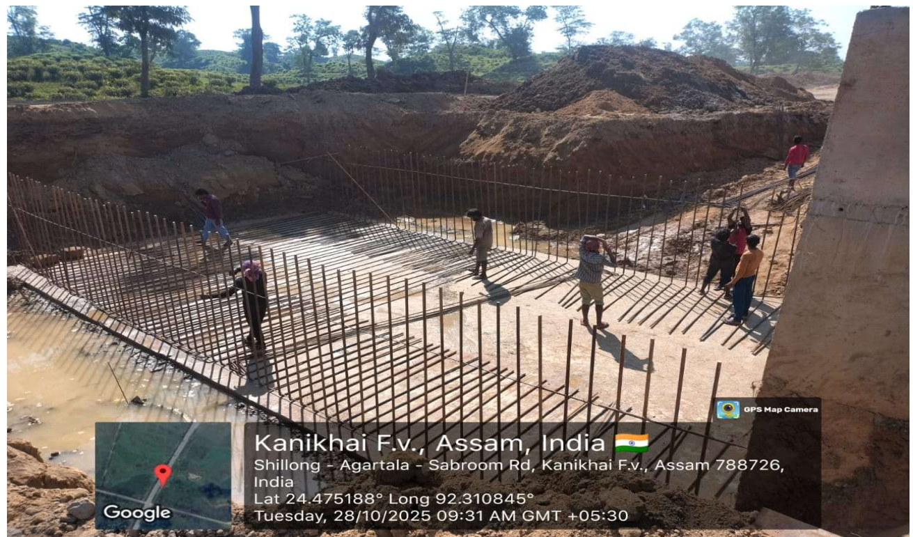
Reinforcement placing work at 98+634 (MNB)
