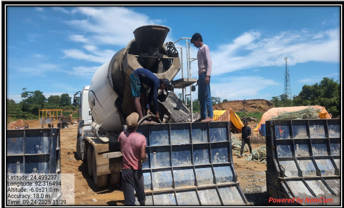
Friction slab casting work in Progress at Ch.- 95+350
