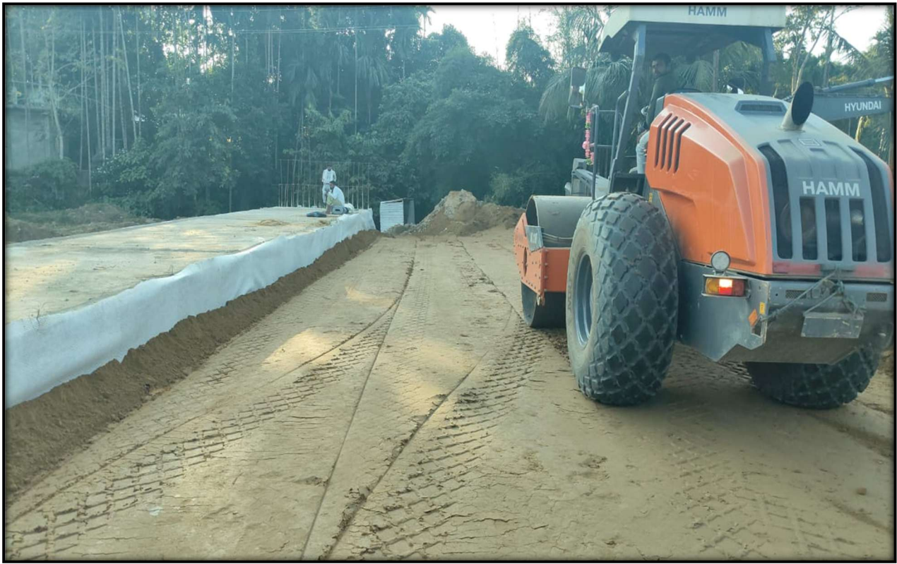
Box-culvert backfilling work at chainage-92+862 A1
