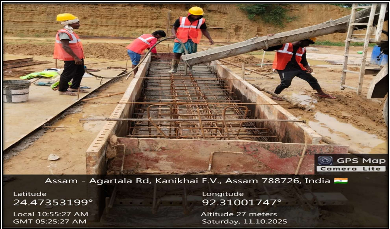
Plank casting for MNB slab-98+631
