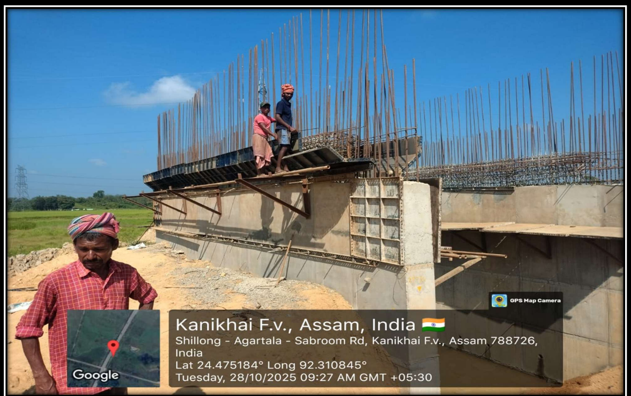
Formwork for Super-structure at chainage-98+508 (MNB)
