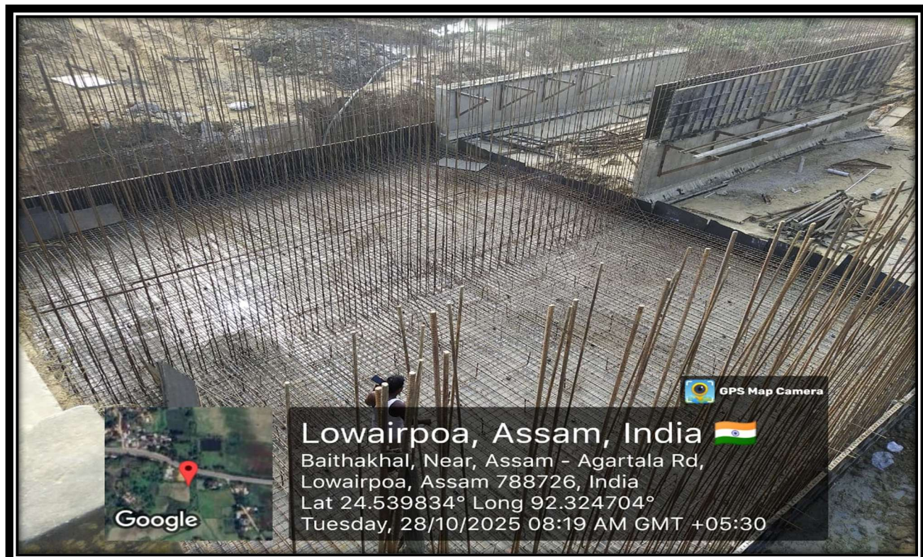
Reinforcement work at chainage-90+543(MNB)
