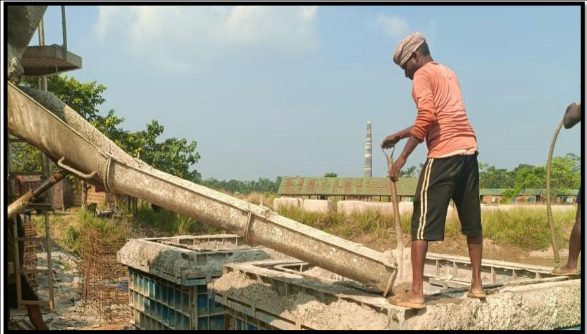
Pre Cast Segment Casting at 0+341
