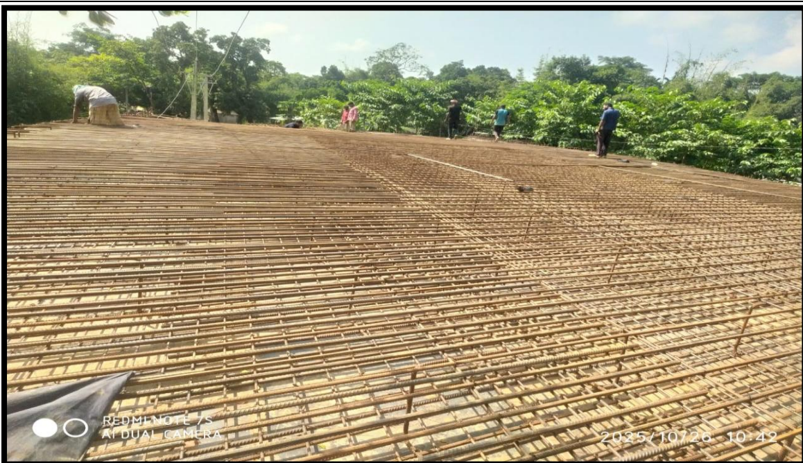
Deck slab Reinforcement work in progress at 9+332 LVUP
