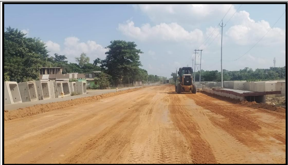
Subgrade Top in Progress at 13+190 To 13+370 LHS
