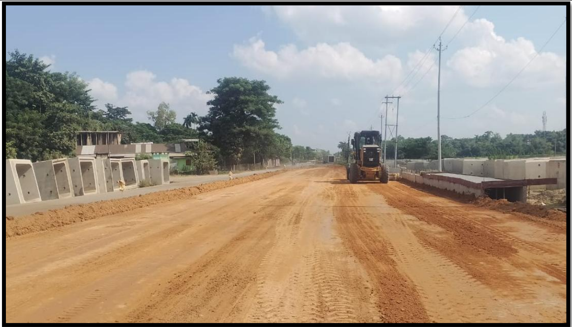
Subgrade Top in Progress at 13+190 To 13+370 LHS
