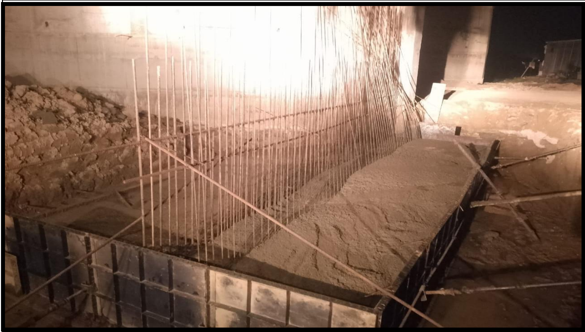
Retaining Wall (Raft) In Progress at 10+098 LVUP
