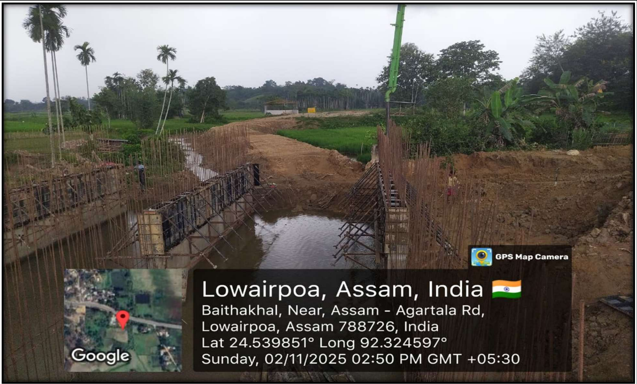
Concrete Pouring work at chainage-90+543(MNB wall)
