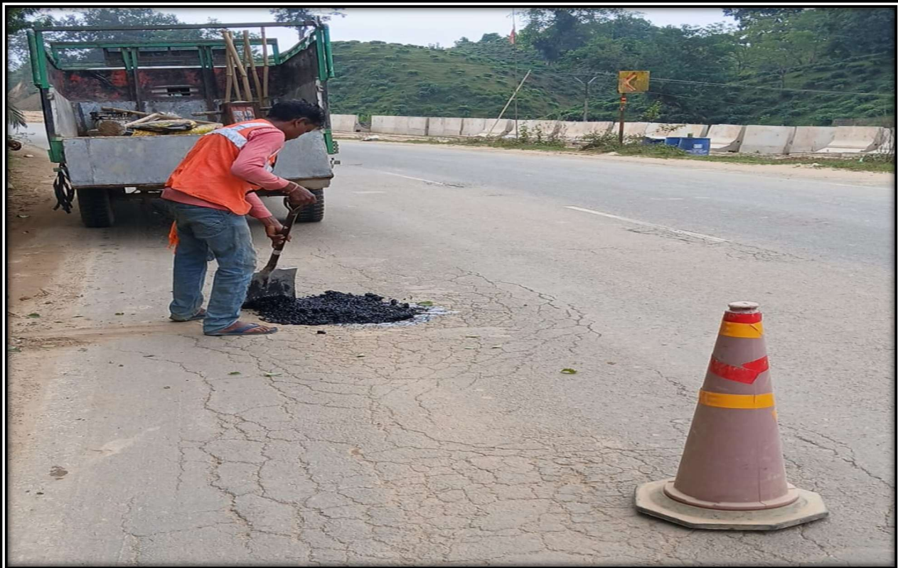
Existing road maintenance work at chainage 89+600
