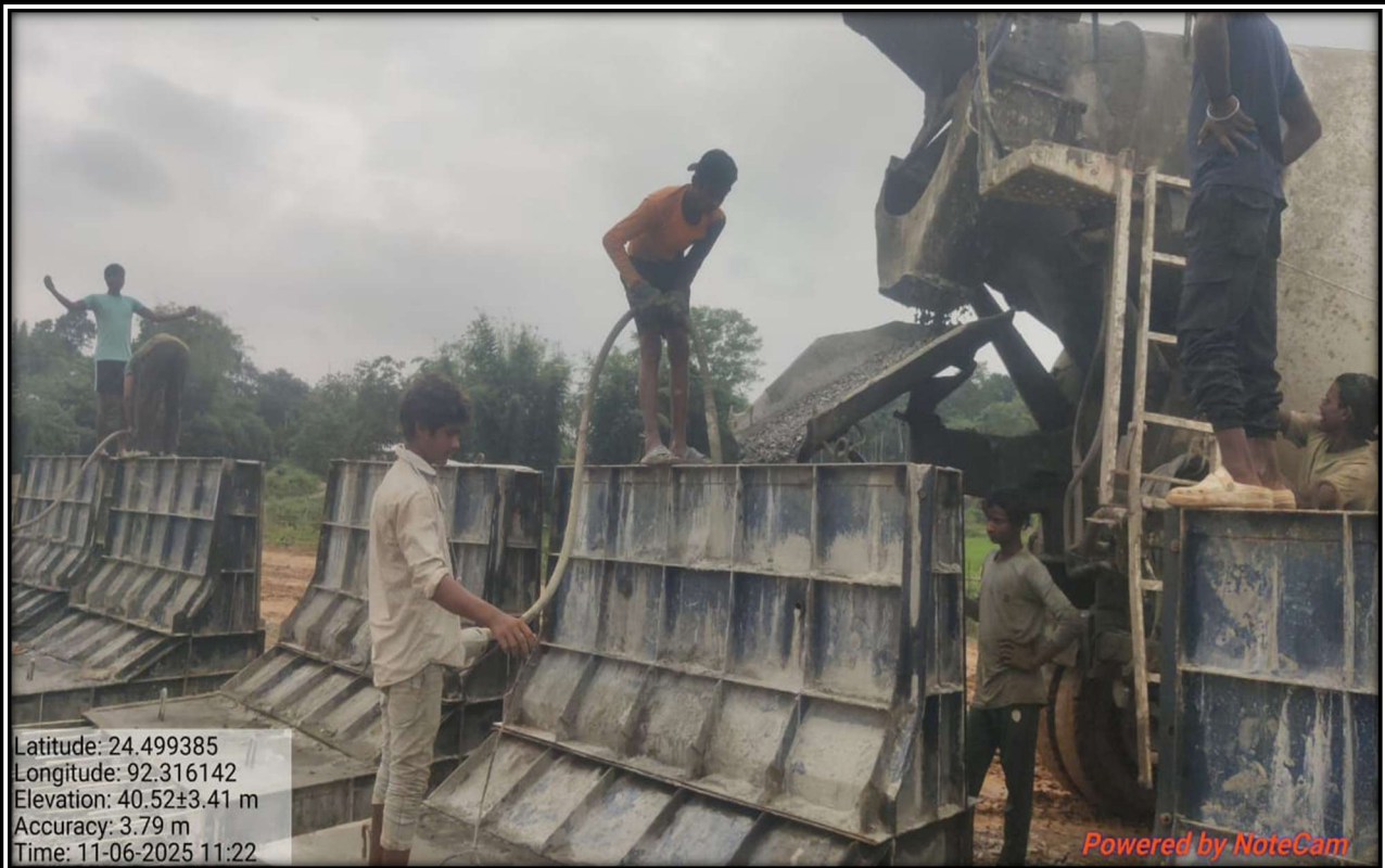
FSCB casting work in Progress at Ch.- 95+350
