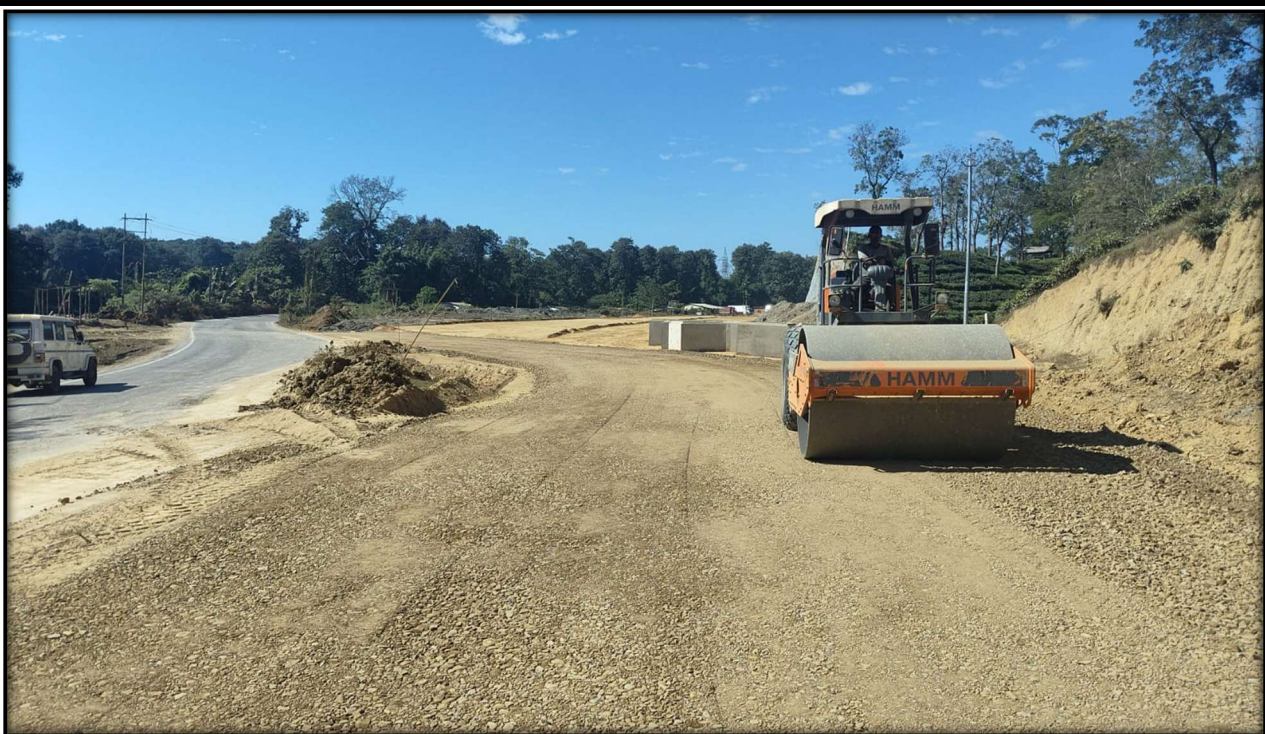
Diversion preparation work at chainage-101+380 (LHS)
