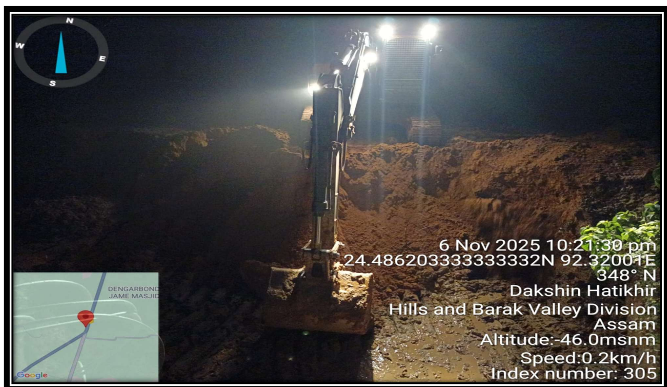
Excavation work atch-96+951 (Box-culvert)
