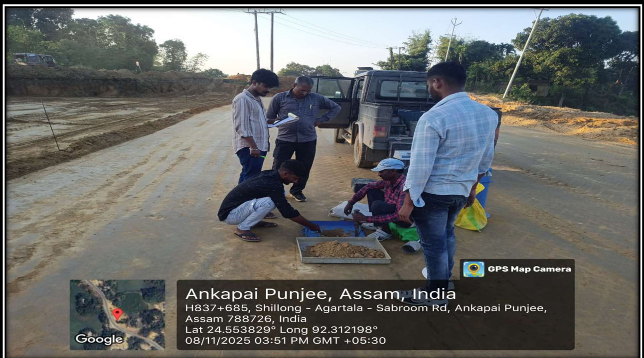
FDD checking of subgrade at chainage-88+500 (BHS)
