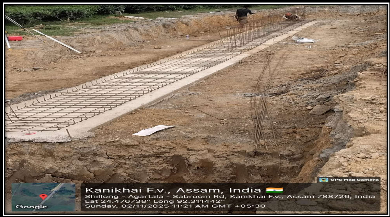
Reinforcement Placing work at chainage-98+300 (Toe wall)
