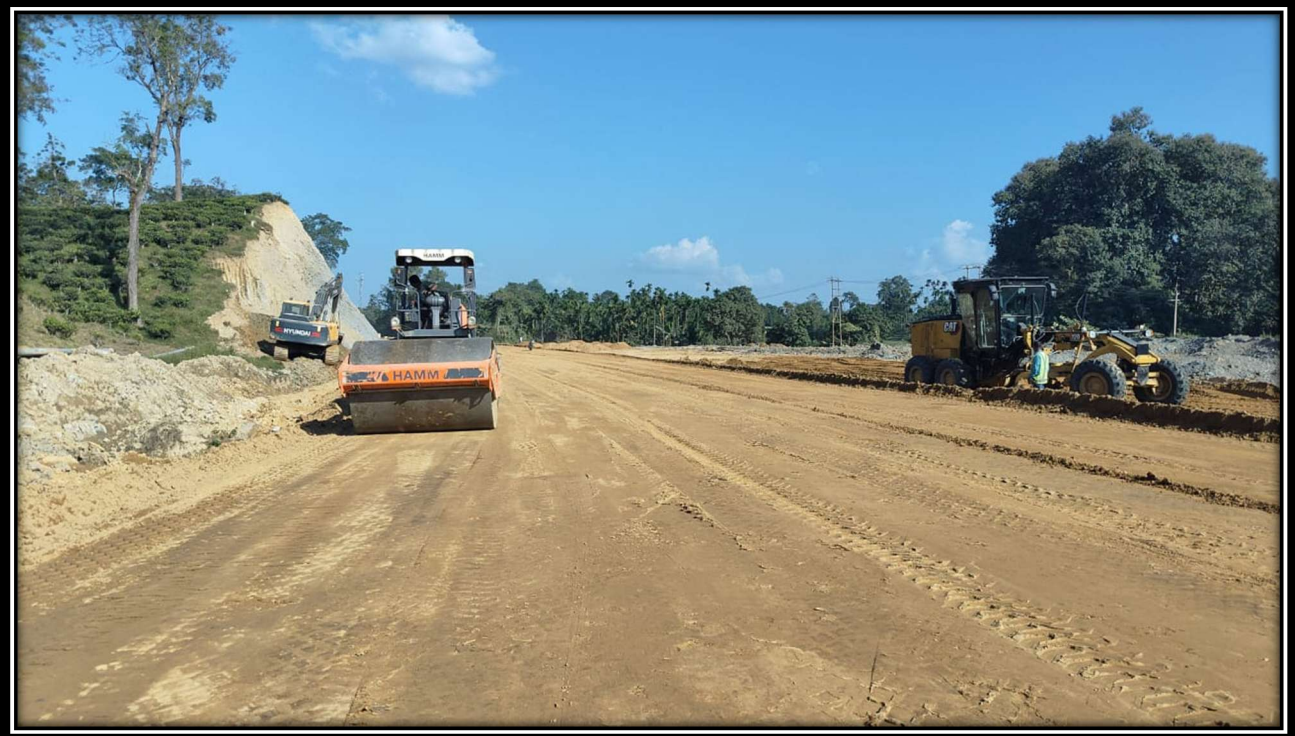
Subgrade rectification work at chainage-101+500(RHS)
