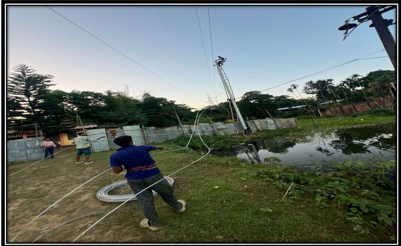
Utility shifting work at chainage-94+200
