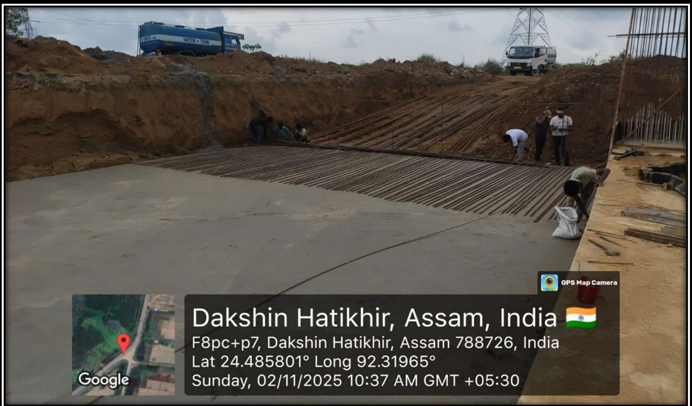
Reinforcement Placing work at chainage-97+000(VUP)
