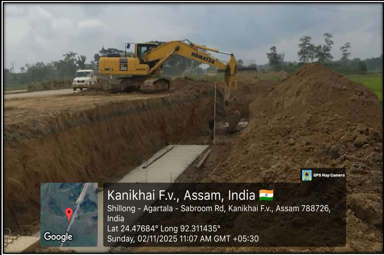
Excavation work for Toe wall at chainage-98+370 (RHS)
