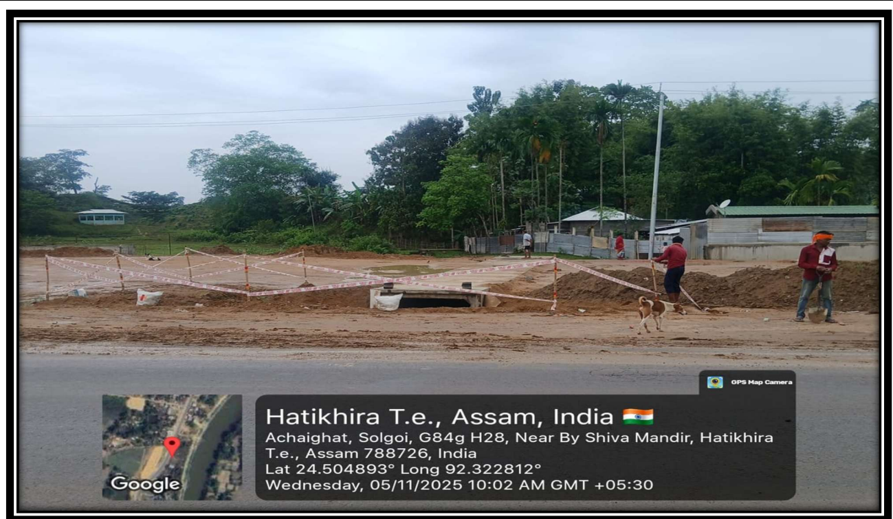
Barricading work at chainage-94+814
