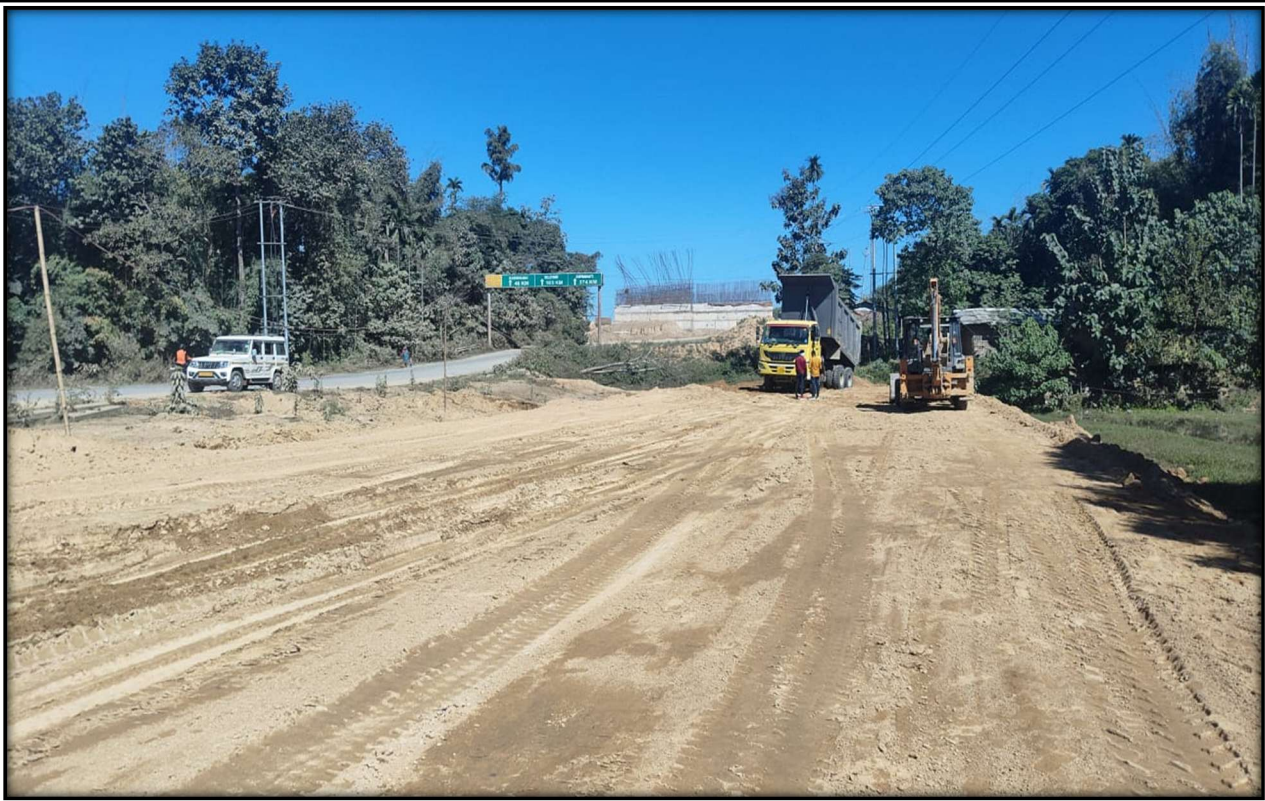
Soil filling work at chainage for 100+400 (PVD work.)
