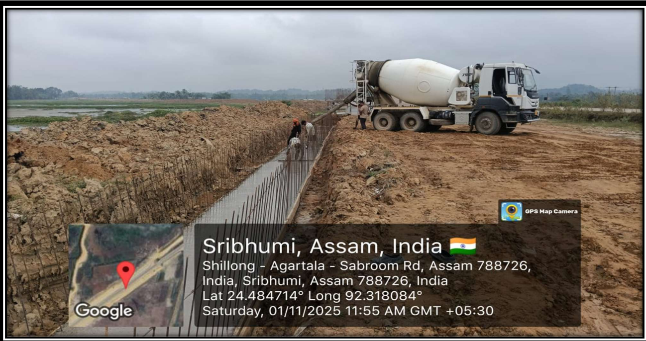
Concrete pouring work at chainage-97+200 (RCC line drain )
