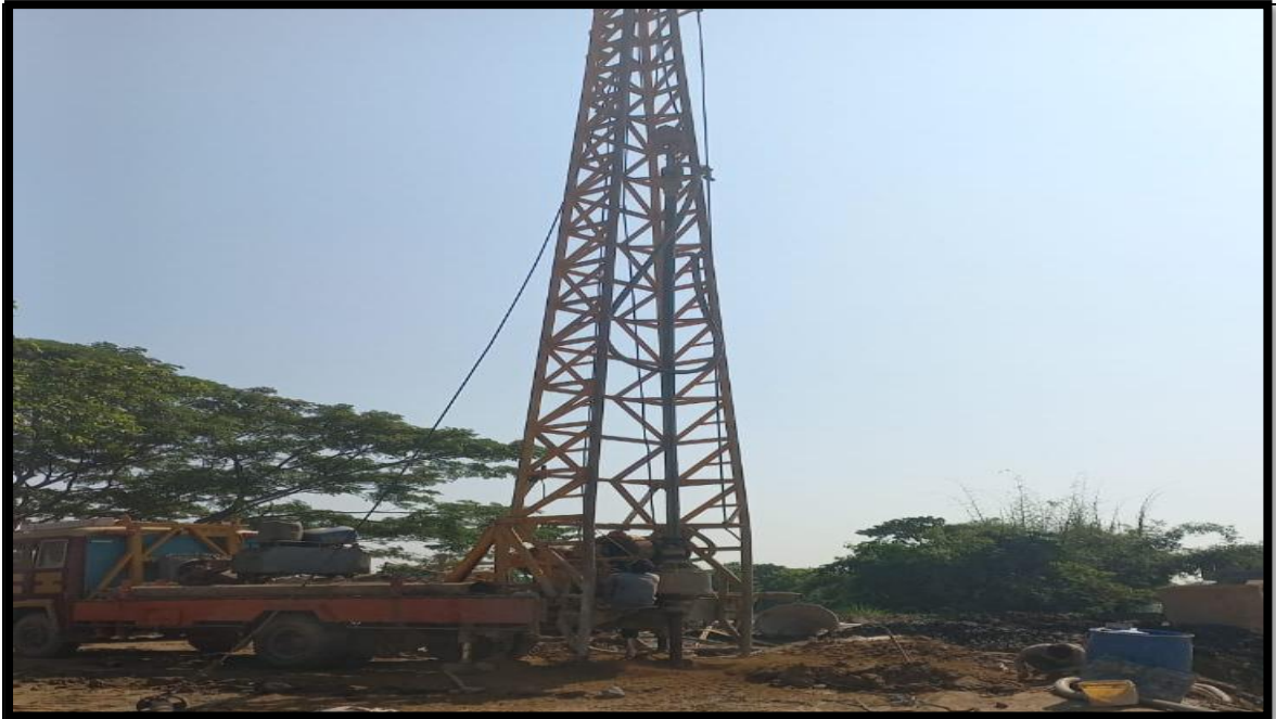
Piling Work in Progress at 2+893 MJB
