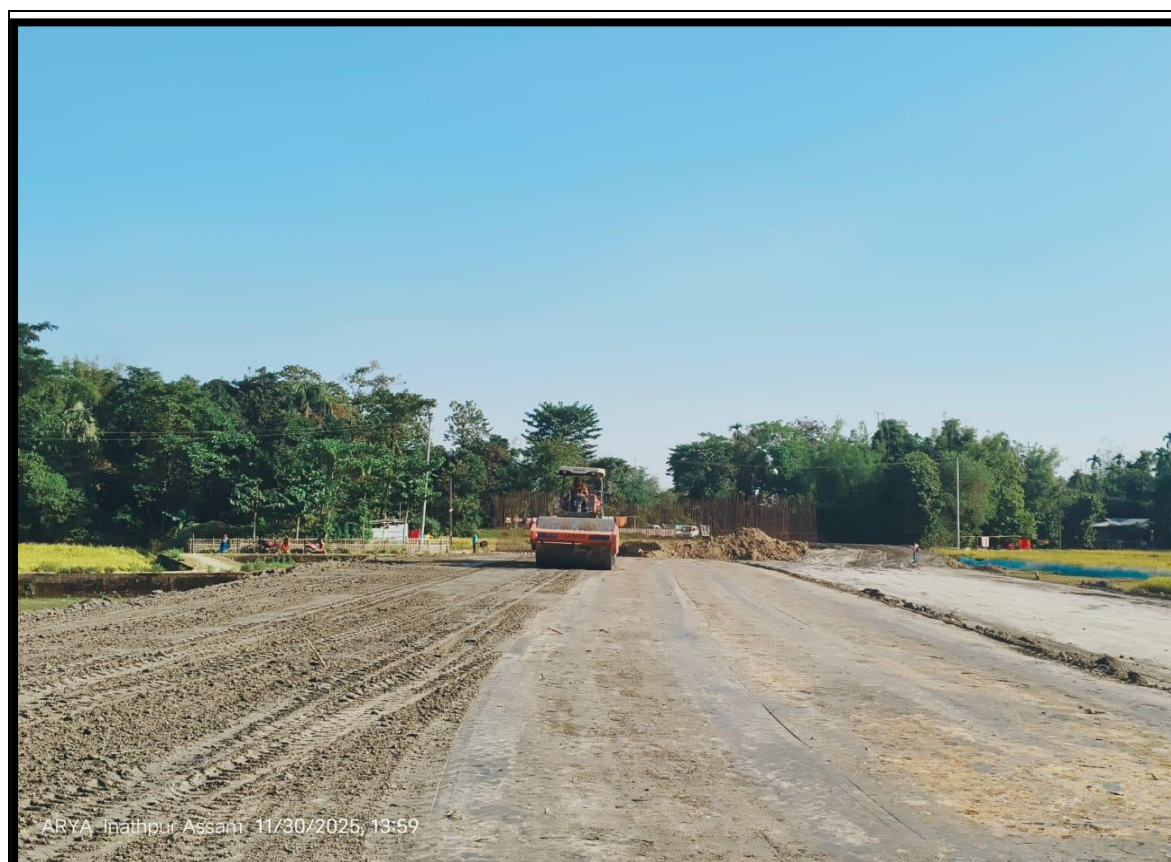
Embankment Layer in Progress at 3+700 To 3+800 BHS
