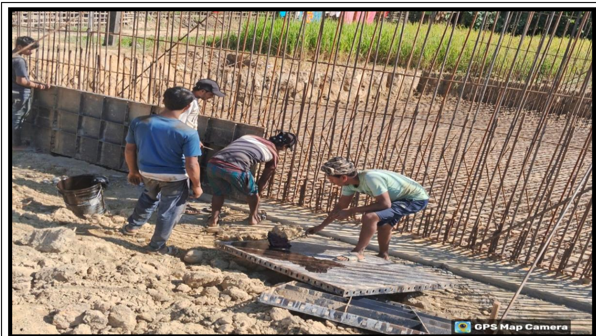
3+728 SVUP Foundation Reinforcement Work In Progress
