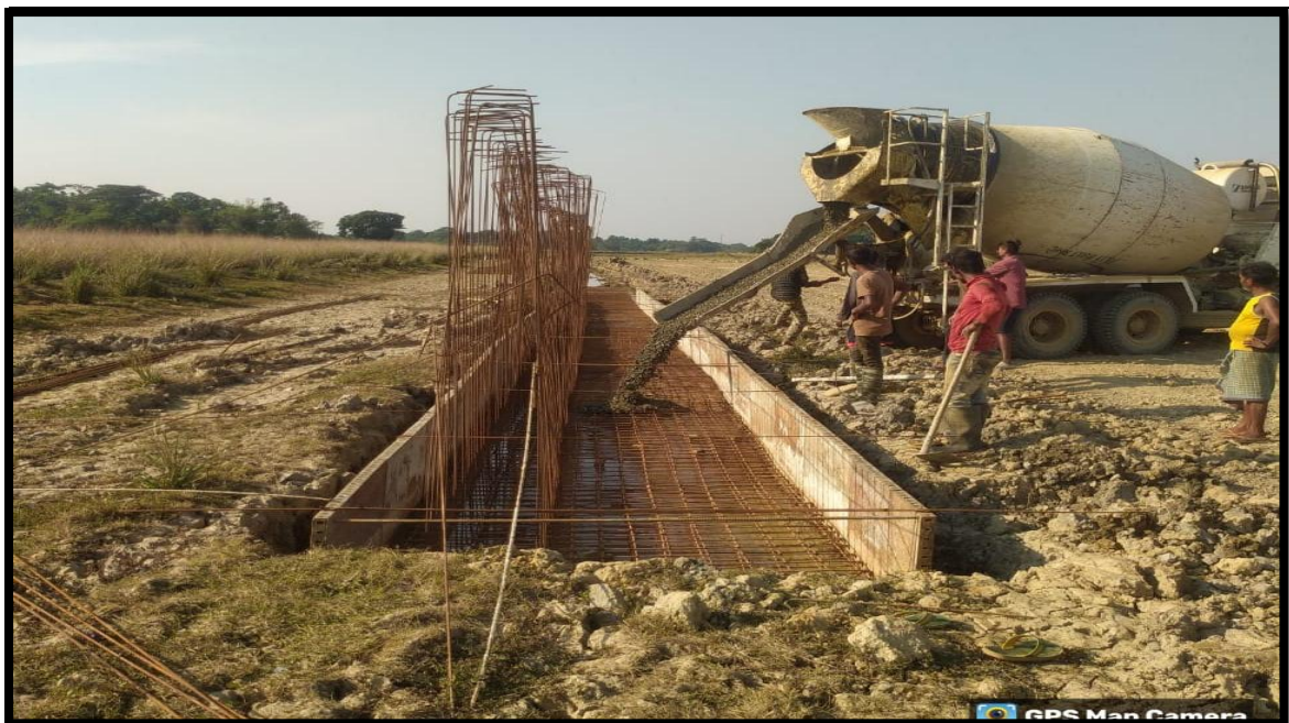
Toe Wall (Raft) In Progress at 2+200
