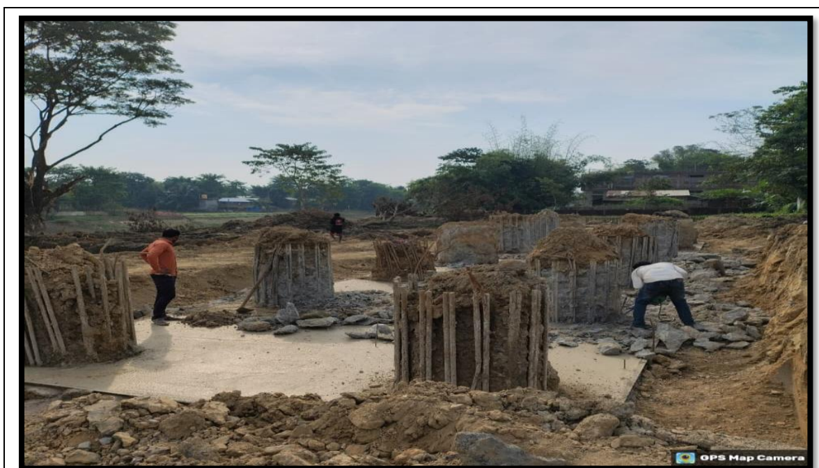
MJB Pile Chipping in Progress at 2+893 MJB
