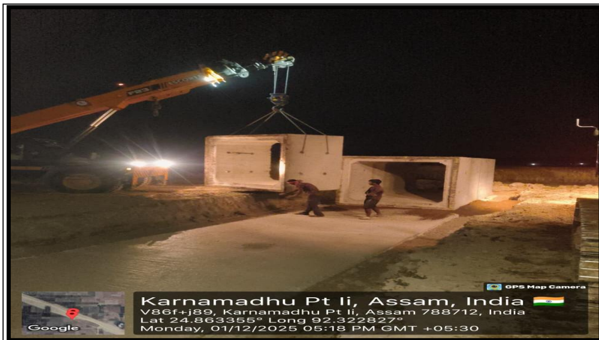
BOX Culvert Segment Erection work in Progress 5+920 BHS
