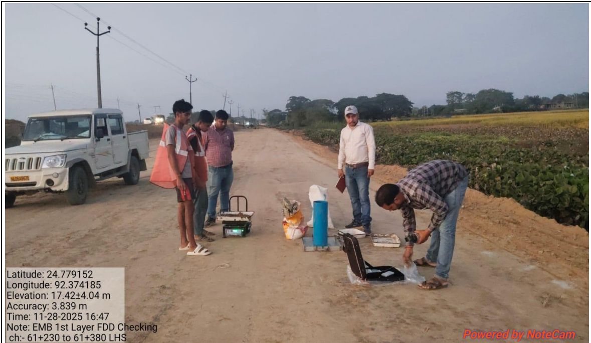
FDD Checking of Embankment Layer 61+230 To 61+380 RHS
