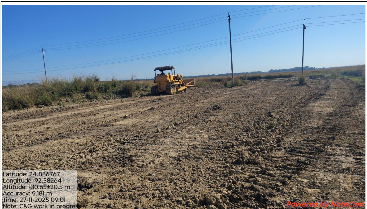
C&G Work in Progress at 52+750 LHS
