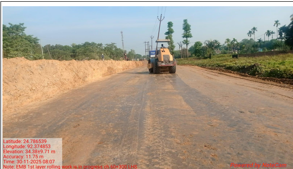
Embankment Layer in Progress at 60+300 To 60+400 LHS
