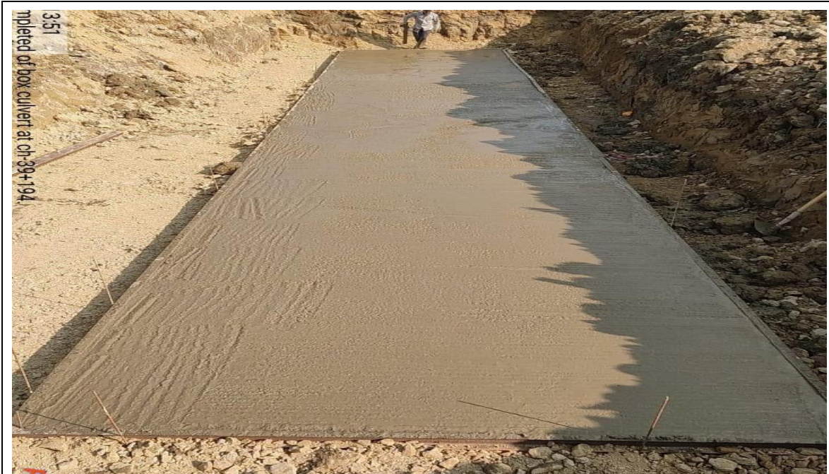
BOX Culvert PCC Complete at 39+194 BHS
