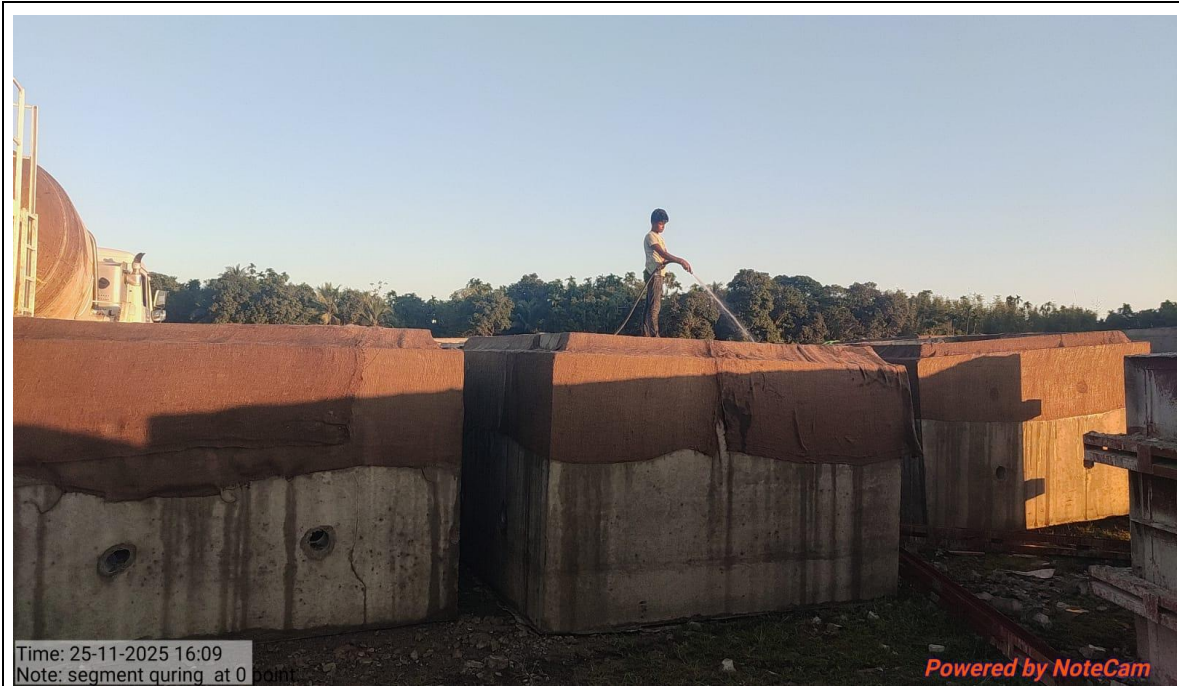
Box Culvert Segment Curing in progress 39+000
