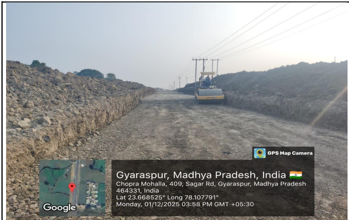
Ch-89+600 LHS RE-Wall leveling Pad Rolling Work in Progress
