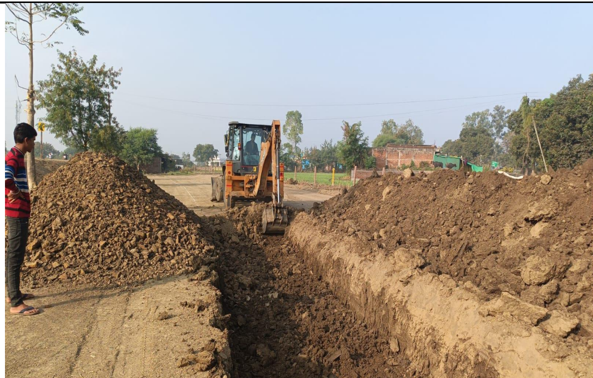
Toe Wall Excavation work in Progress at Ch. 100+620
