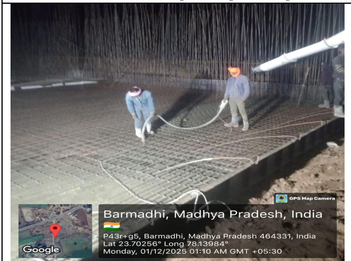
LVUP Raft Concrete Pouring Work in Progress at ch. 94+875 LHS
