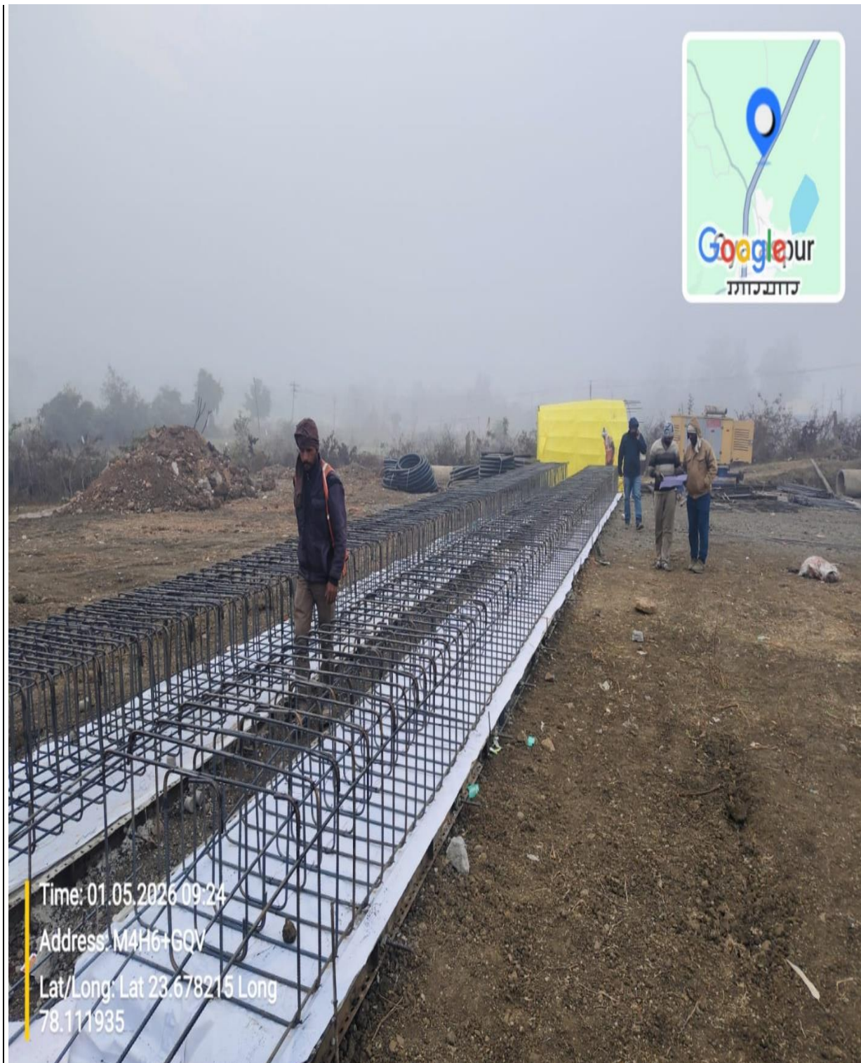
Ch 90+540 VUP precast beam reinforcement binding in progress
