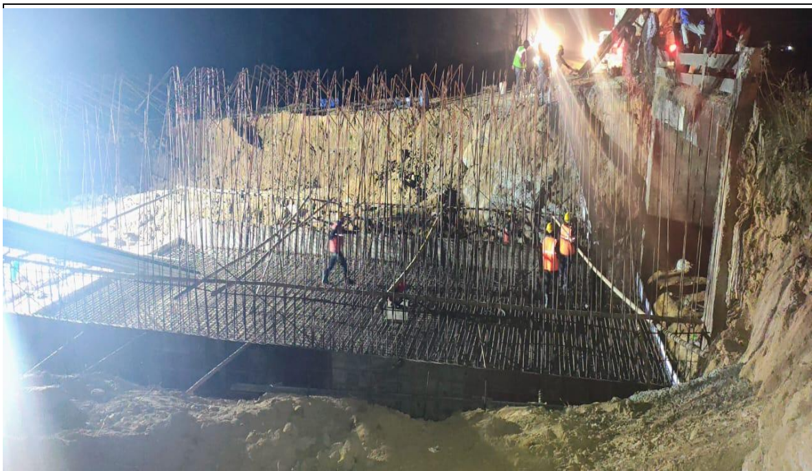
58+103 MNB Foundation LHS Concrete Pouring In progress
