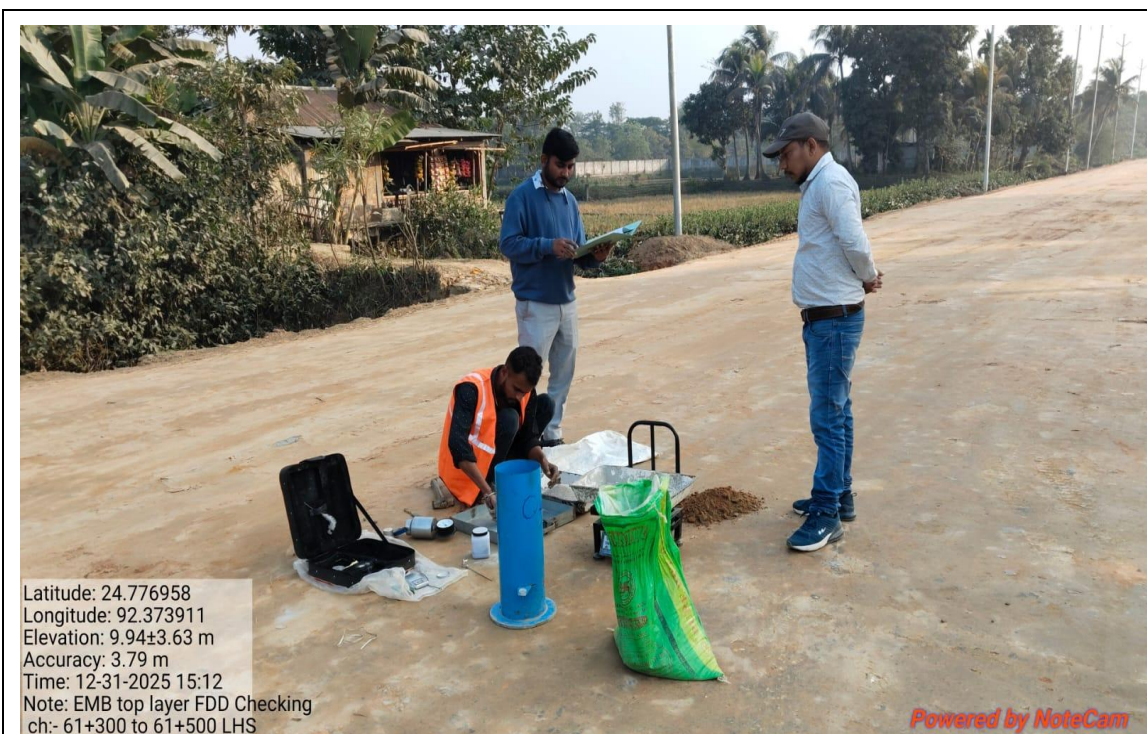
EMBANKMENT TO FDD CHECKING FDD at 61+300 To 61+500 LHS
