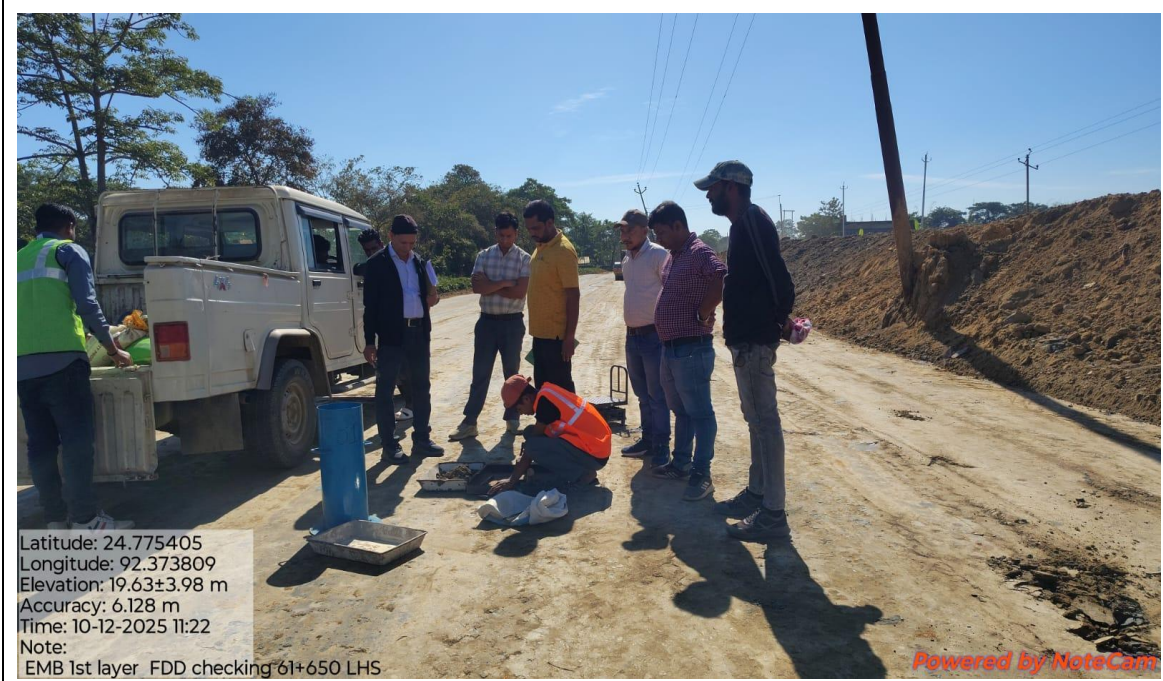
Embankment 2 nd layer in progress 61+500 To 61+700 LHS
