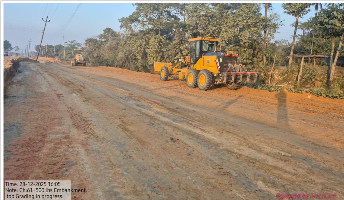
Embankment Layer in progress 61+200 To 61+500 LHS
