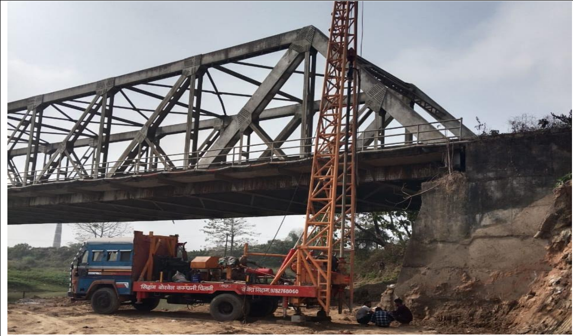
Abutment Pilling Work in progress 54+560 MJB
