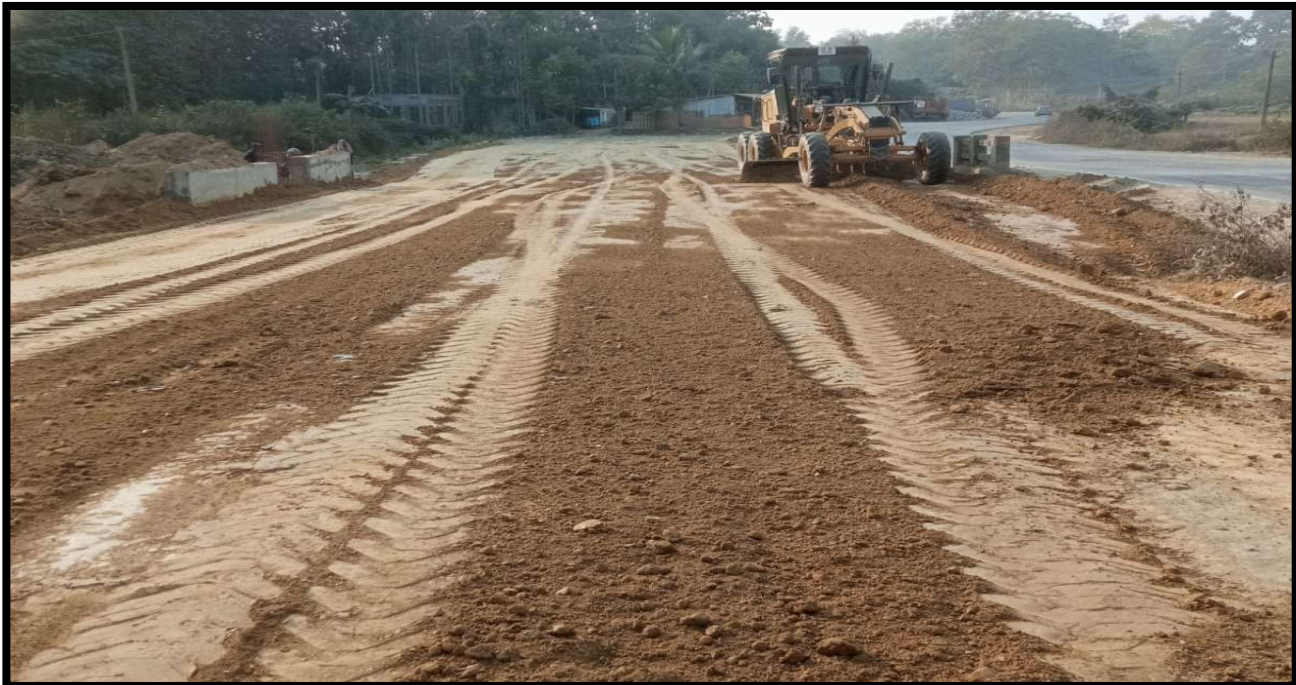
Sub-Grade top at chainage-101+860 to 101+930 LHS MCW
