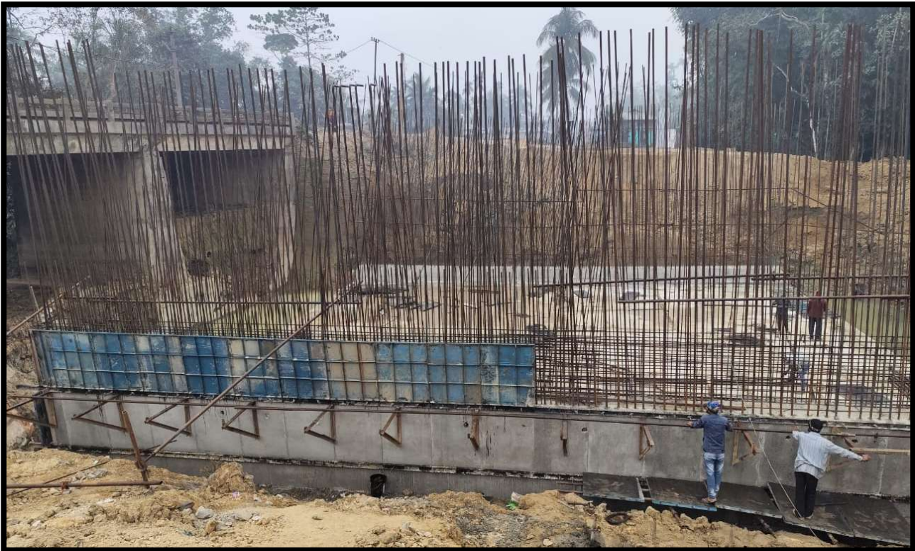
Wall 2 nd Lift casting for MNB at Ch-95+595 RHS
