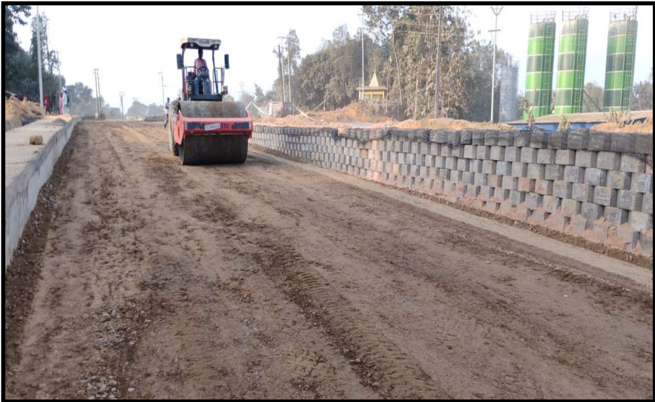
Service Road GSB work at chainage-88+870 RHS
