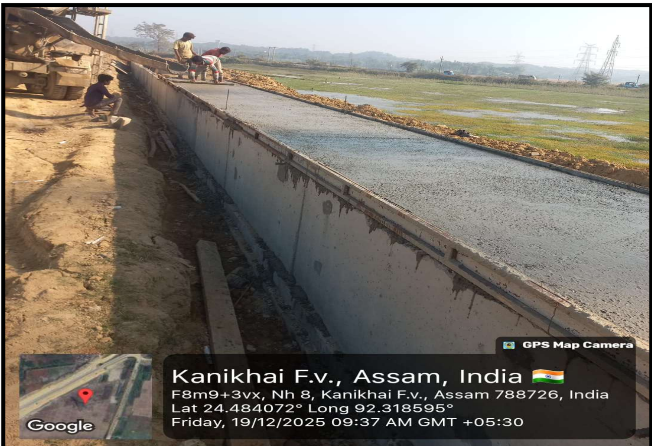
Drain Slab at Ch-97+212
