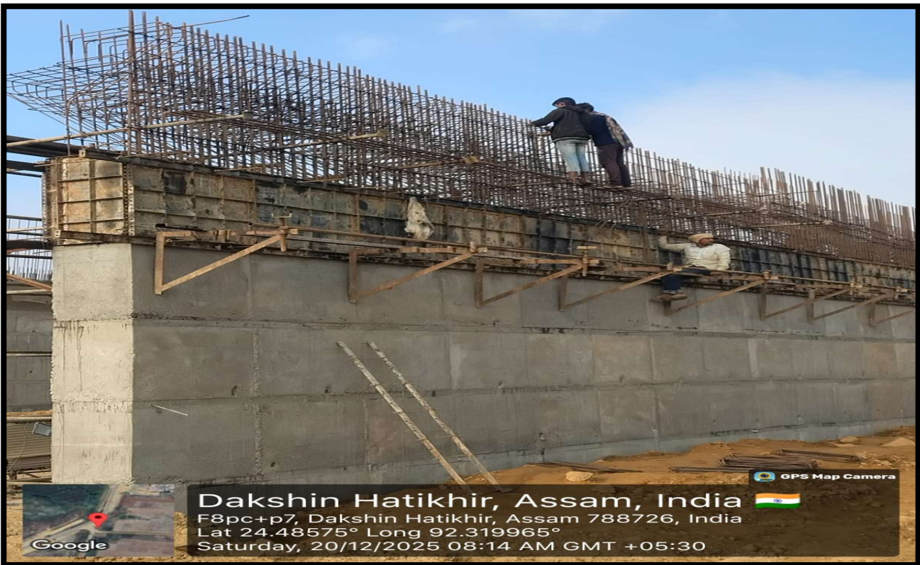
Bracket work at 97+000 VUP
