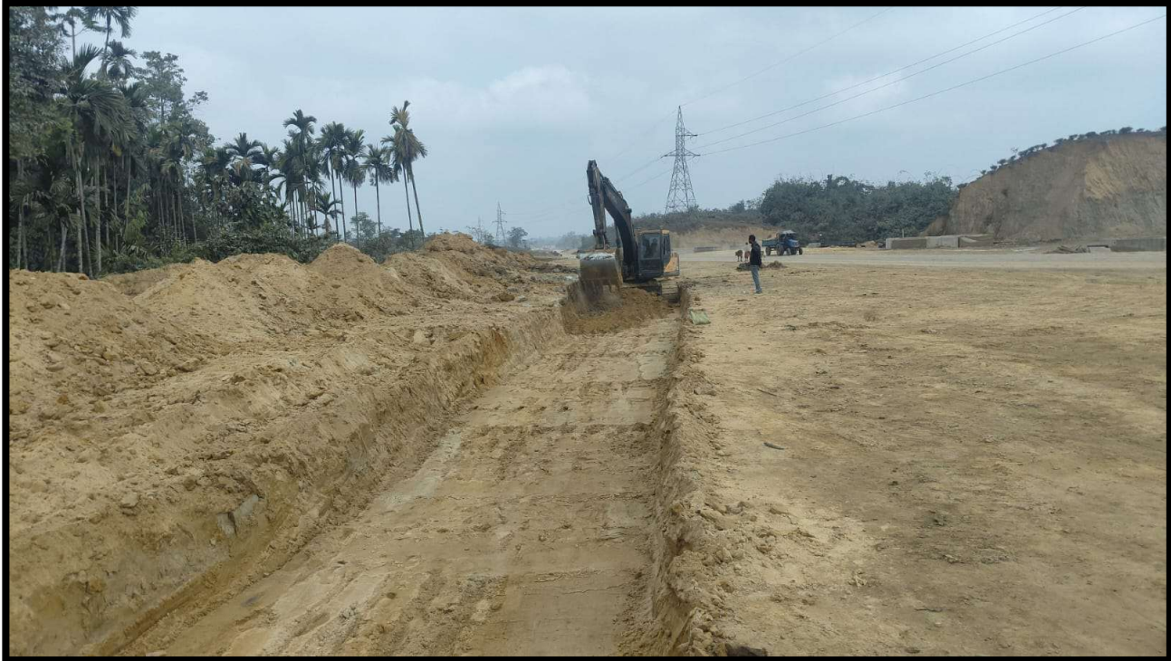
Drain Excavation Work in Progress
