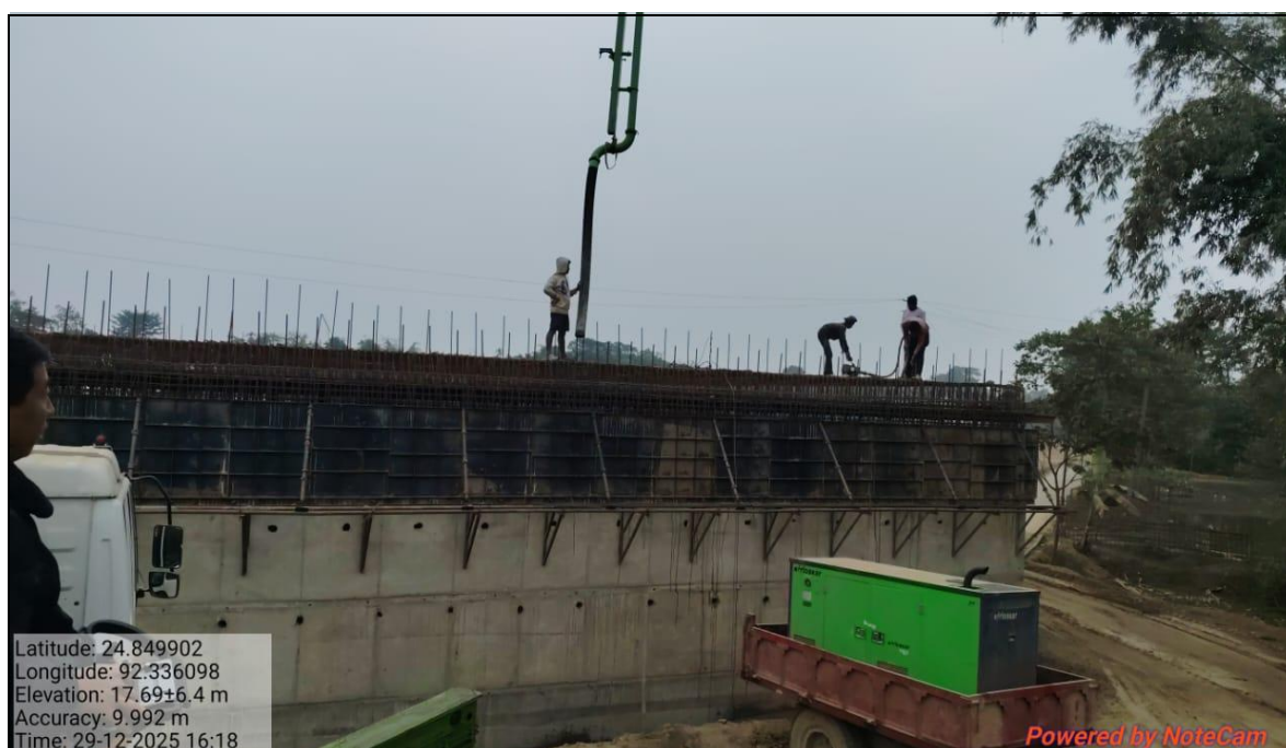
3+886 LVUP 3rd Lift Concrete Work In Progress
