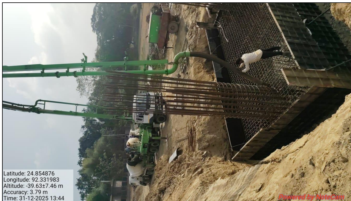
ROB A1 Abutment Pile Cap in Progress at 4+624 ROB
