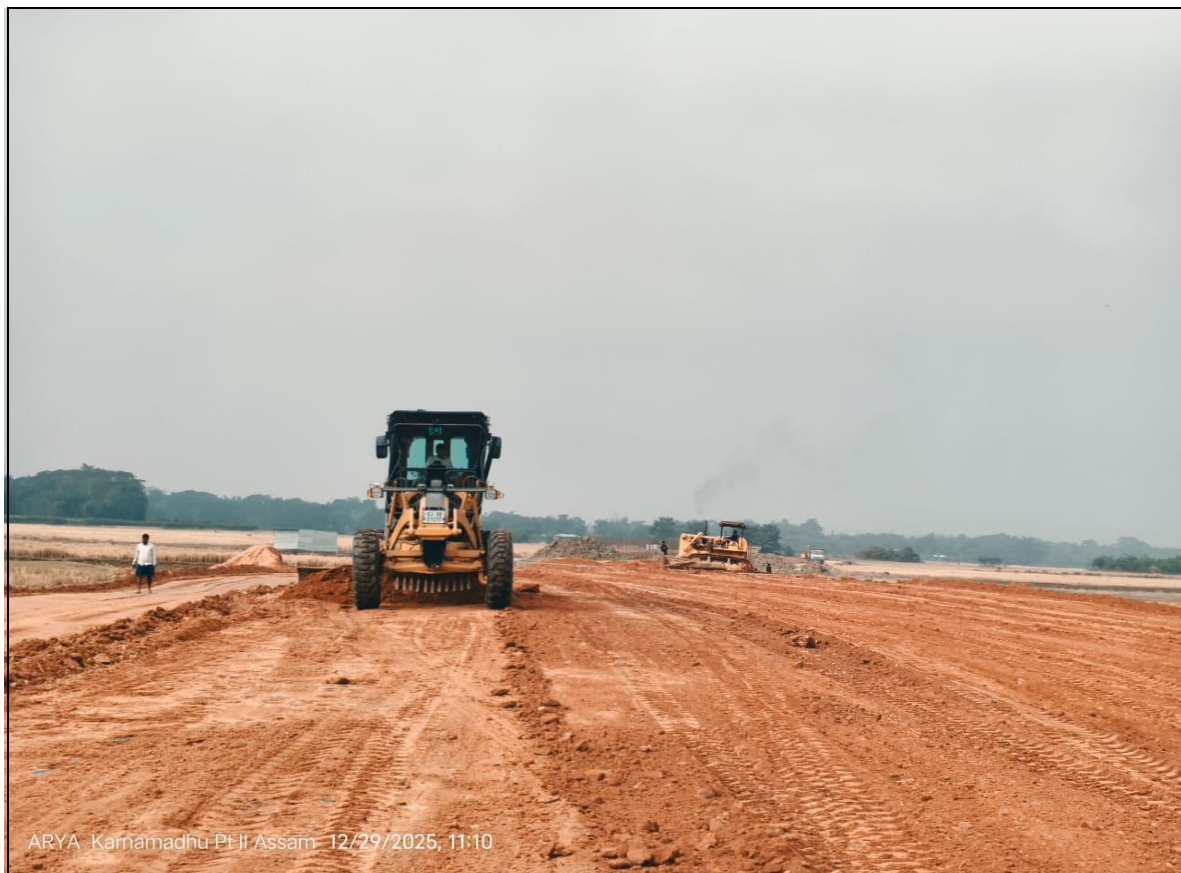
Embankment Layer in Progress at 6+020 To 6+180 BHS
