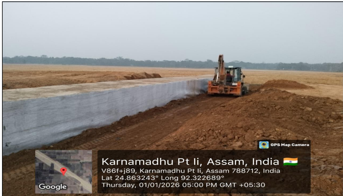
BOX Culvert Backfilling work in Progress 5+920 BHS
