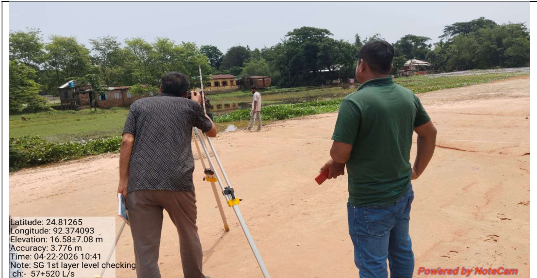
SUB GRADE TOP LAYAR CHECKING WITH IE REPRESENTIVE
