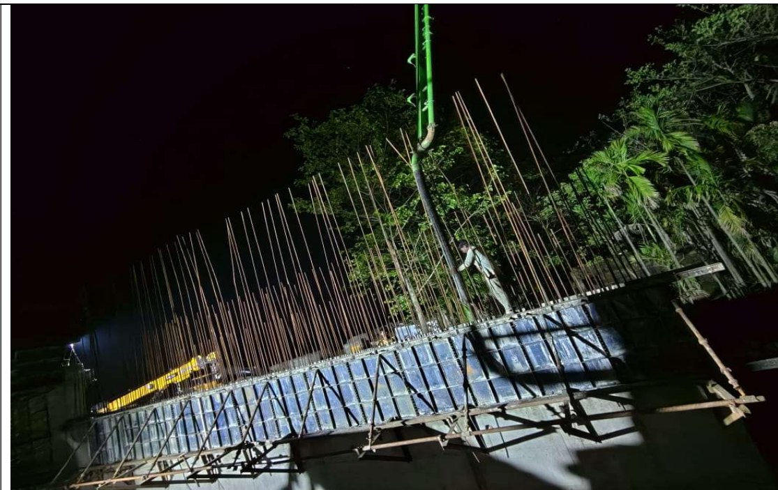
42+800 LVUP A1A2 LHS WALL 2 ND LIFT CONCRETE WORK IN PROGRESS
