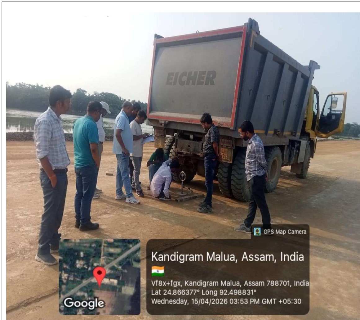
FIELD CBR TEST CONDUCT WITH IE TEAM AT CH-39+500 BHS
