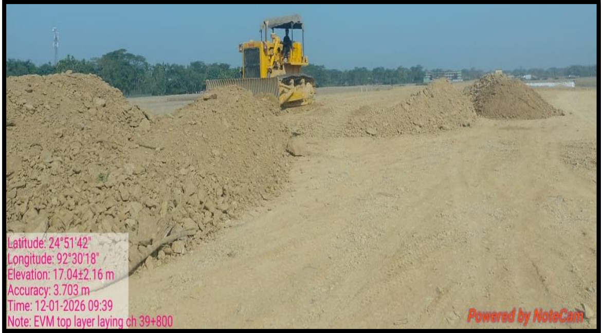
EMB TOP LAYER IN PROGRESS AT CH. 39+800
