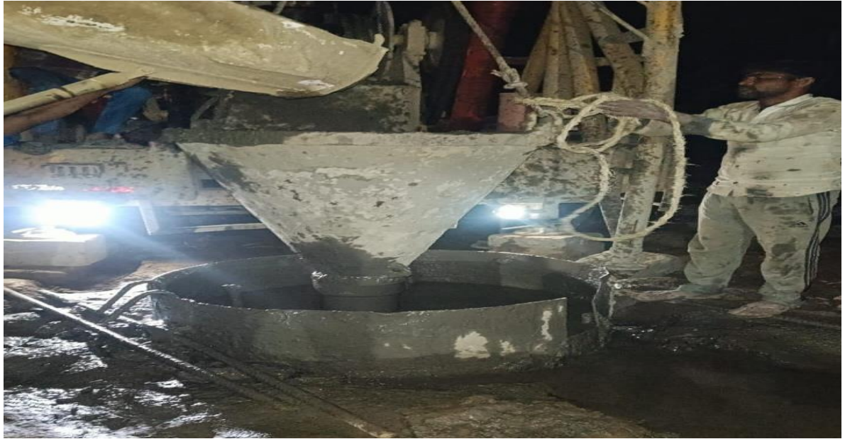
Abutment Pilling Work in progress MJB
