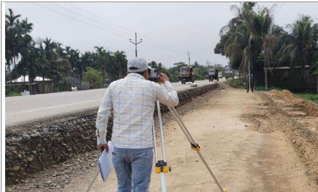
SG TOP LAYER LEVEL CHECKING AT CH. 62+200 TO 62+400 RHS
