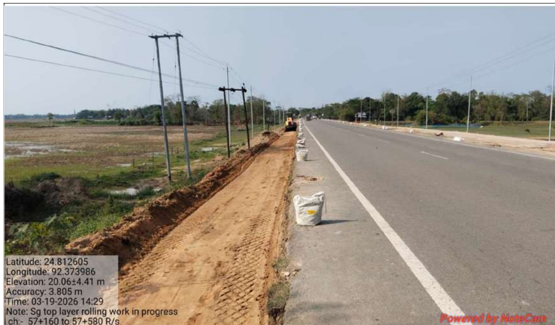
SG TOP LAYER ROLLING AT CH. 57+160 TO 57+580 RHS
