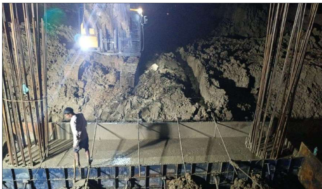
48+557 PILE CAP CASTING
