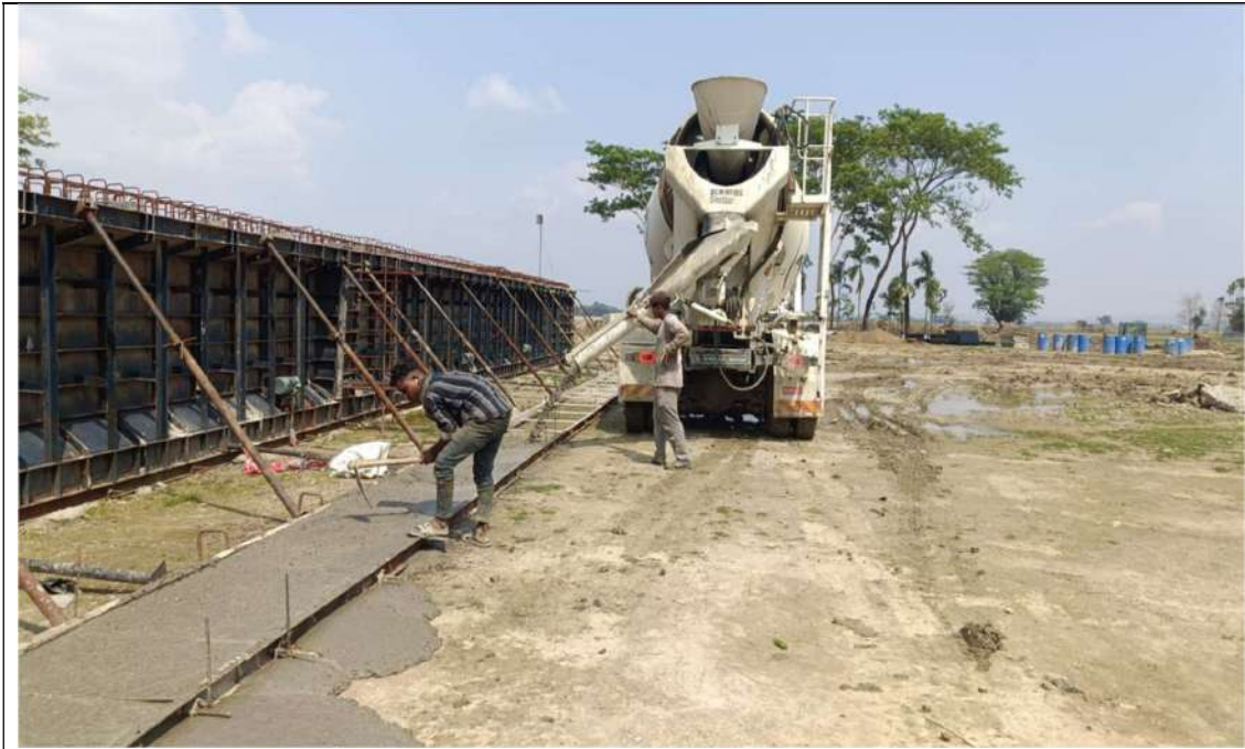
Toe wall raft concrete pouring work in progress AT 55+600 to 55+640 RHS
