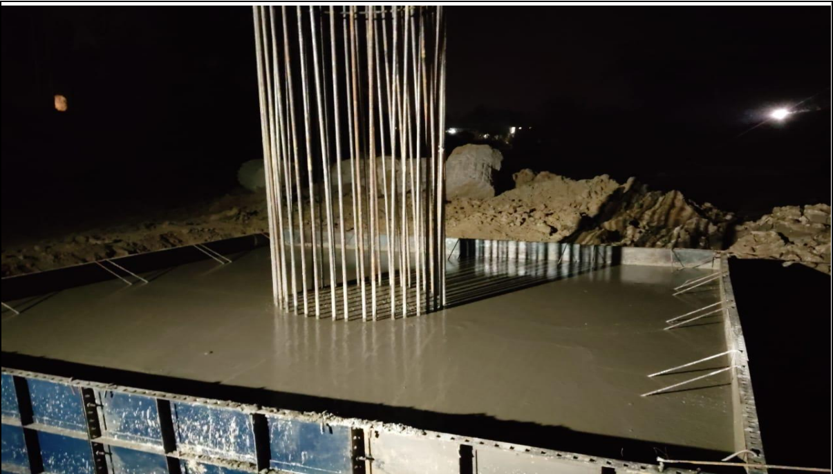
PILE CAP CASTING COMPLETE AT 48+557 P2 RHS
