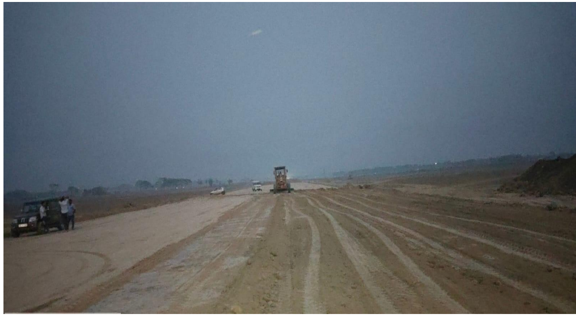
EMB TOP LAYER GRADING WORK IN PROGRESS AT CH. 44+500 LHS
