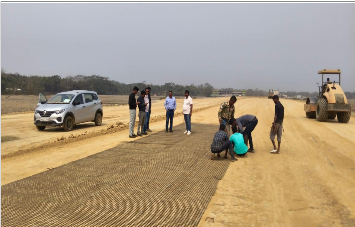
Geogrid laying at 39+600 to 39+700
