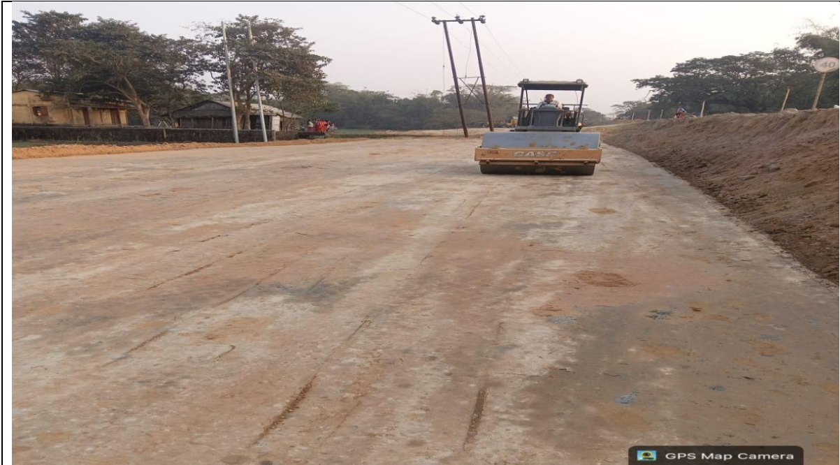
EMB TOP LAYER ROLLING AT CH. 57+300 TO 57+500 LHS
