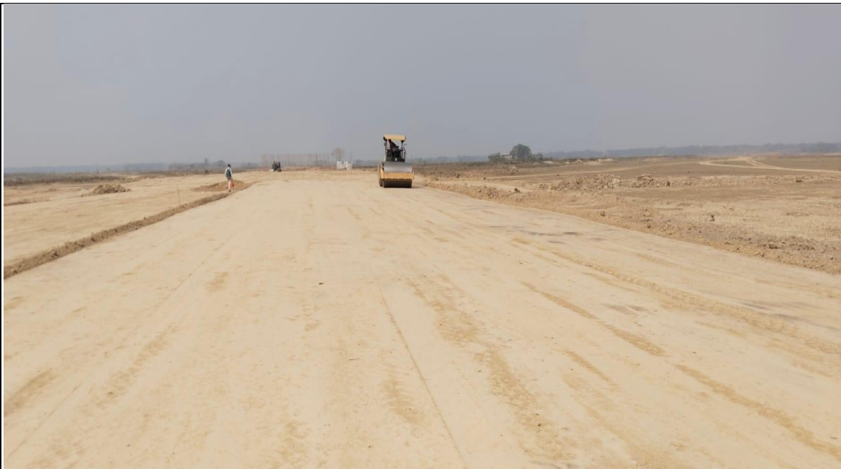
EMB TOP LAYER ROLLING AT CH. 44+000 TO 44+600 RHS
