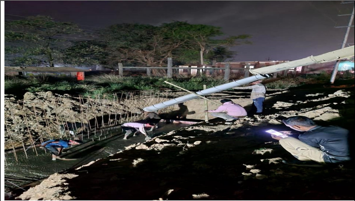
Toe wall raft concrete pouring work in progress AT 55+600 to 55+640 RHS
