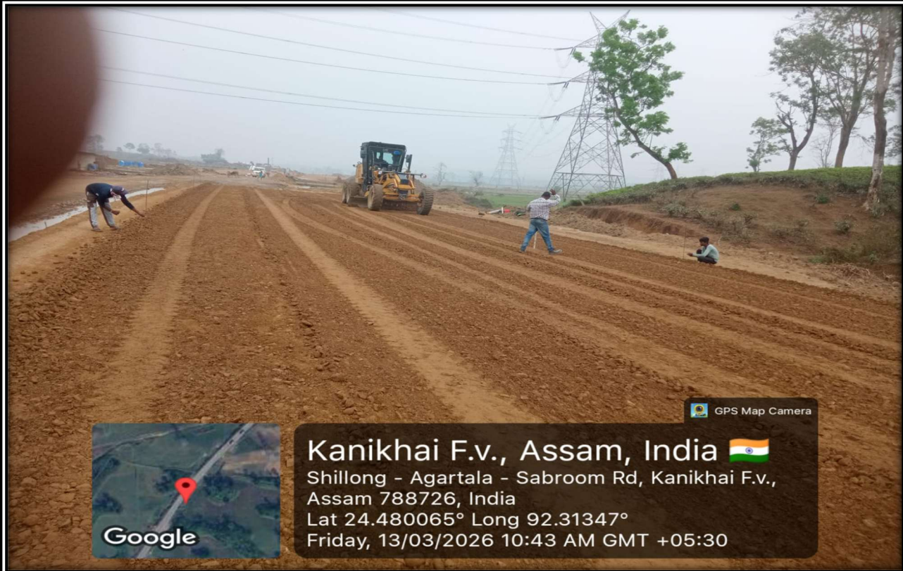
GSB Top Layer work in progress at Ch- 97+850 To 98+010 LHS MCW.
