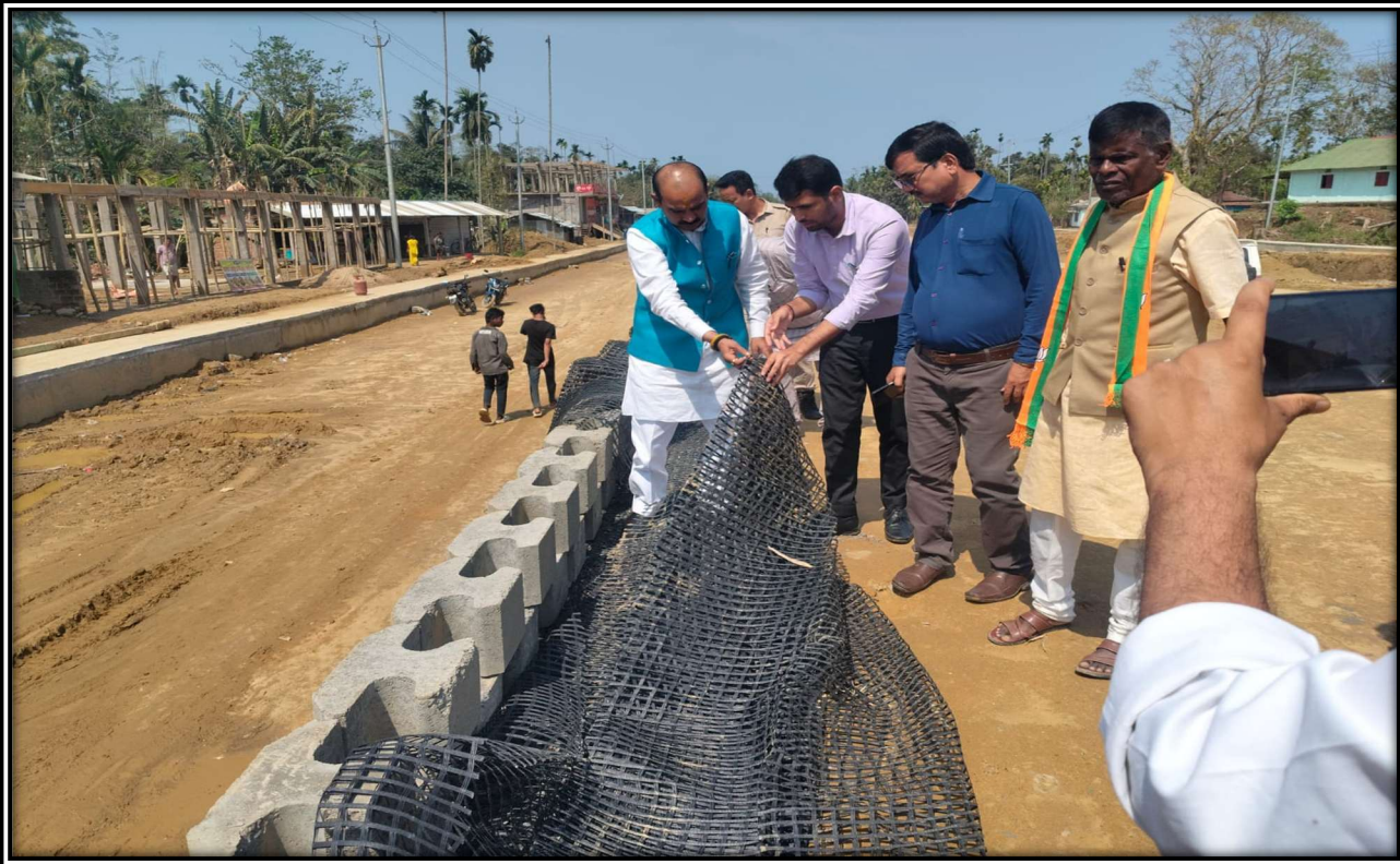
Site Visit, Minister of State, Road Transport and Highway
