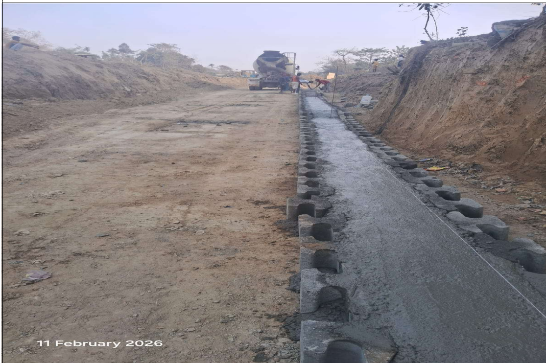
MNB Raft Concrete Pouring In Progress At Ch- 11+351
