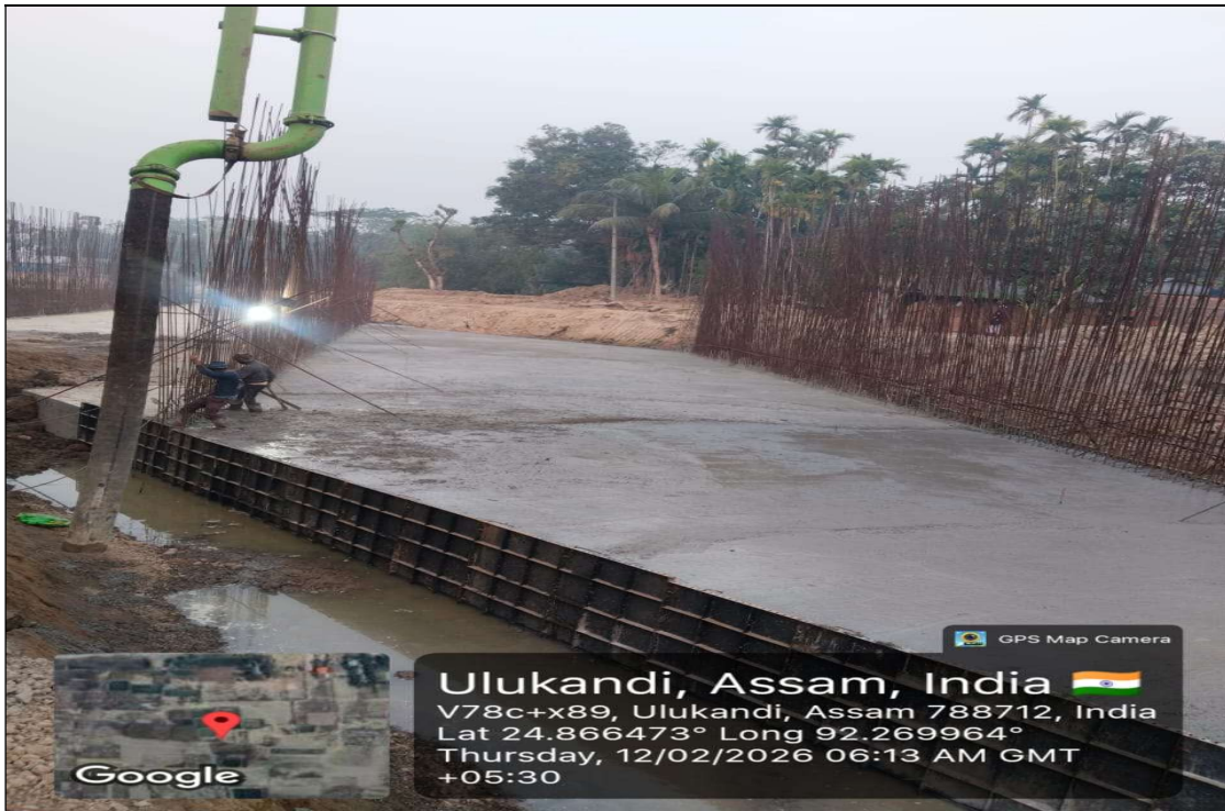
MNB Raft Concrete Pouring In Progress At Ch- 11+351
