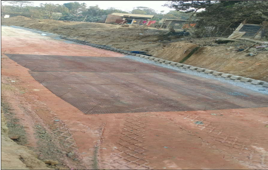
Geo-Grid Laying Work In Progress Ch- 04+200
