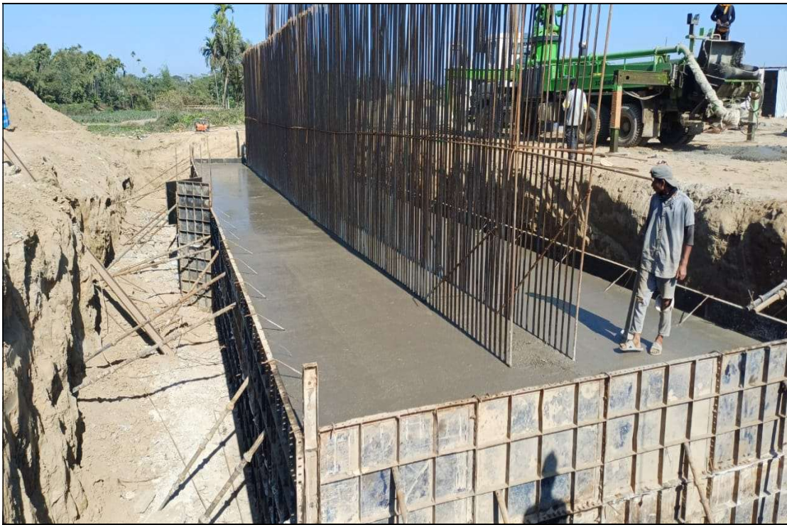
A1 Abutment Cap Concrete Pouring In Progress Ch- 05+332 At MJB
