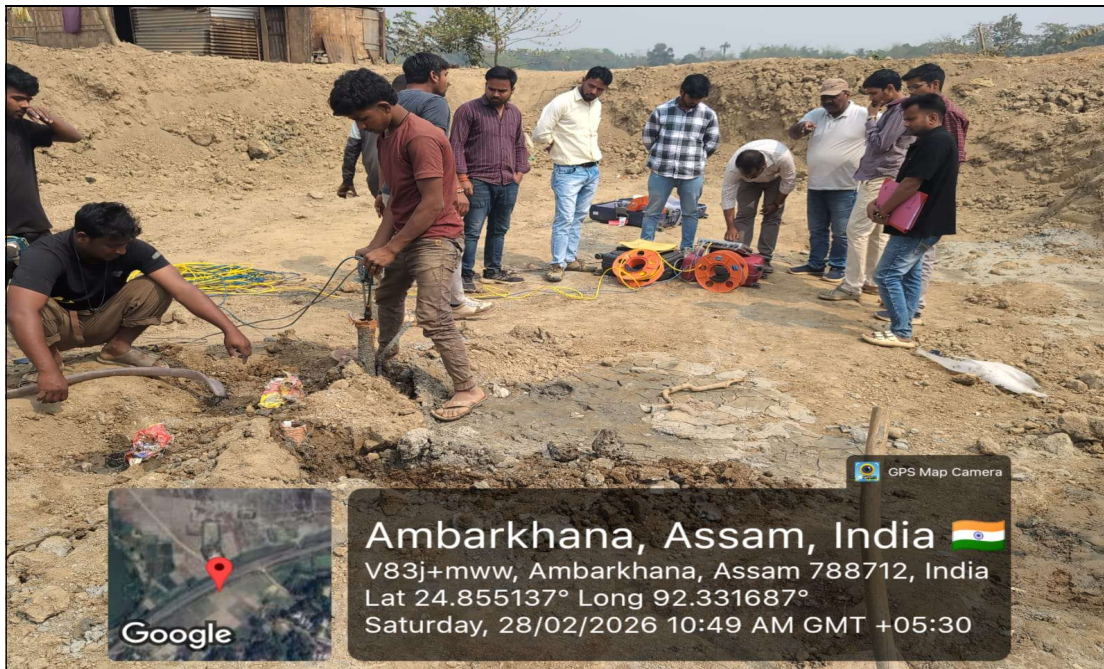
Cross Hole Ultrasonic Monitor(CHUP TEST) In Progress Ch- 04+624 At ROB
