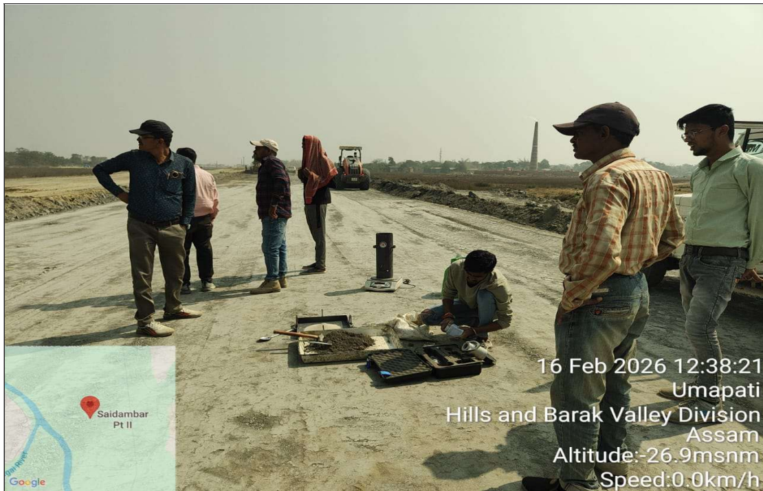
FDD Testing For Embankment Top At Ch- 01+500 To 01+600
