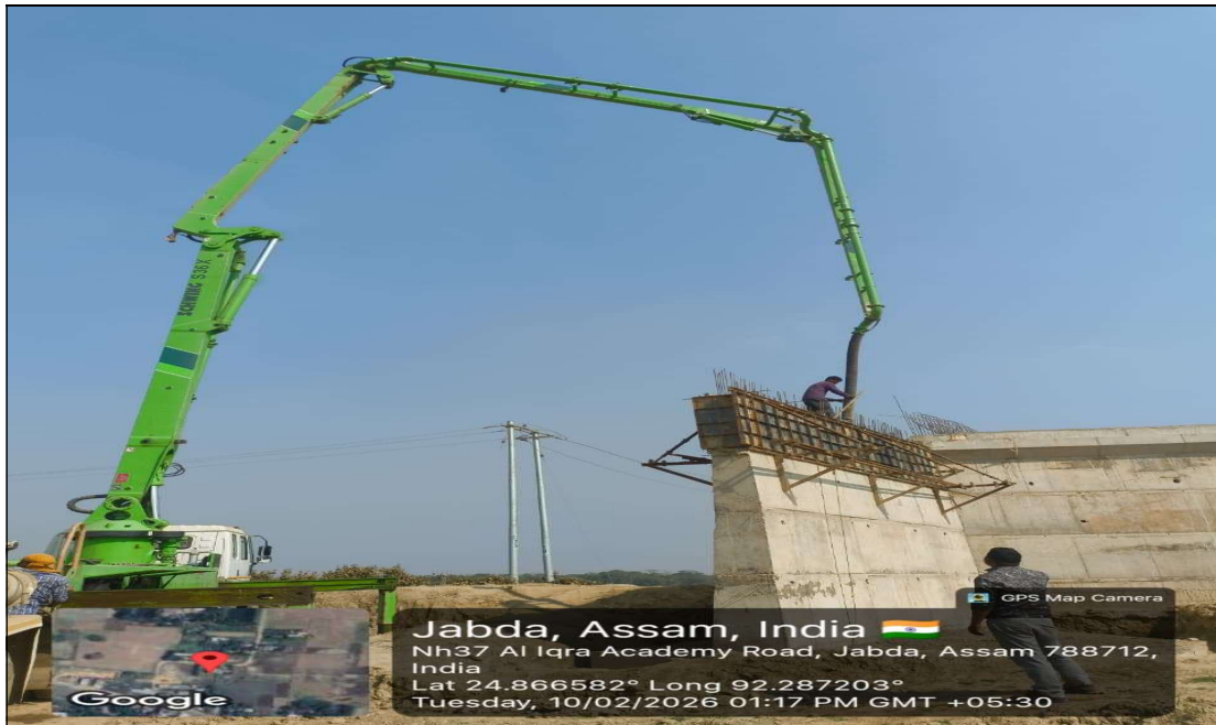
LVUP Final Lift Concrete Work In Progress At Ch- 10+098
