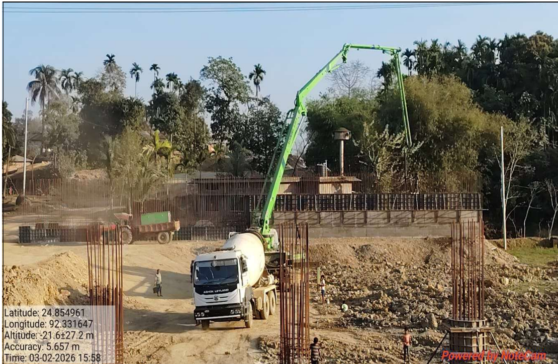
BUP Wall 2 nd Lift Concrete Pouring In Progress At Ch- 04+534
