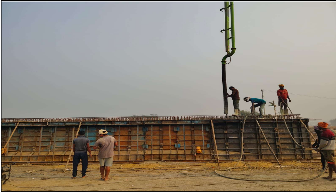
PSC Girder Concrete Pouring in Progress at Ch- 00+526 At MJB
