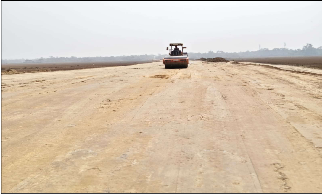
Embankment Layer in Progress at Ch- 06+420 To 06+600 BHS
