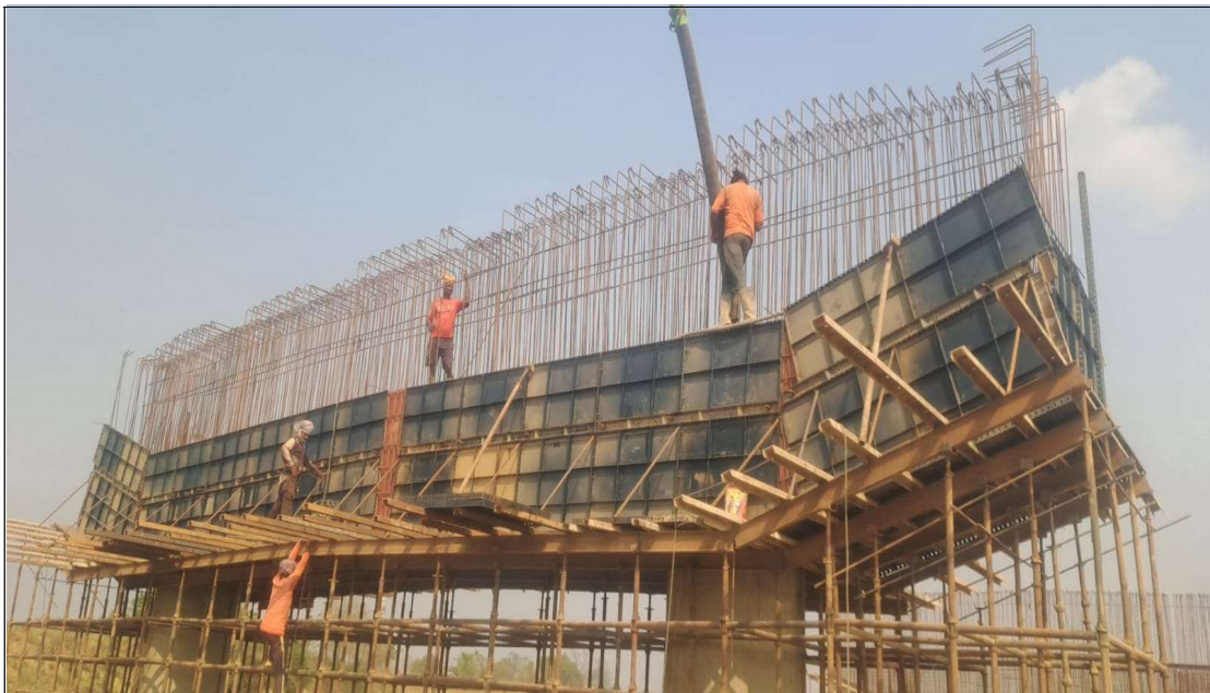
Pier Cap Concrete Pouring In Progress Ch- 00+526 At MJB
