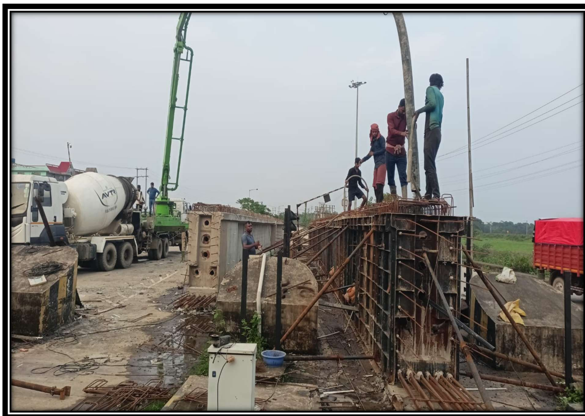
PSC Girder concrete pouring work in progress at Ch.- 42+800
