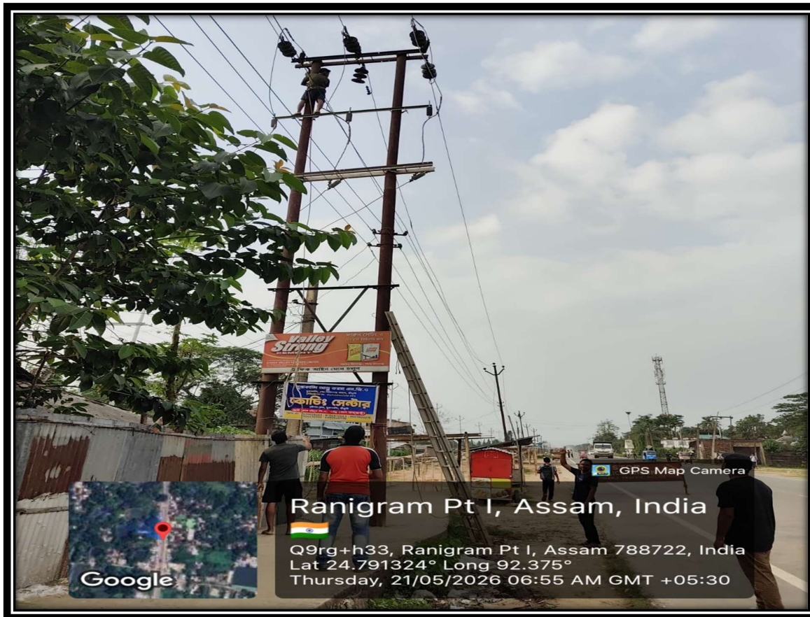
33kv Line dismantling work in progress at Ch.- 59+900 To 61+900
