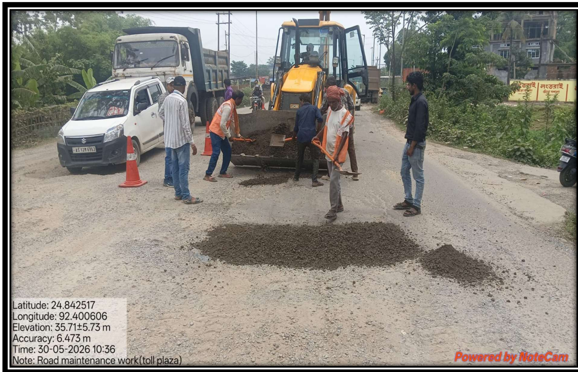
Road maintenance work in progress at toll plaza.
