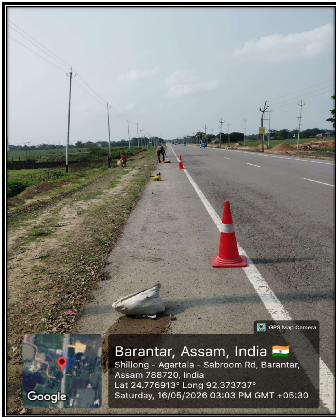
Safety work (Edges protection) work in progress at Ch. 61+500 LHS
