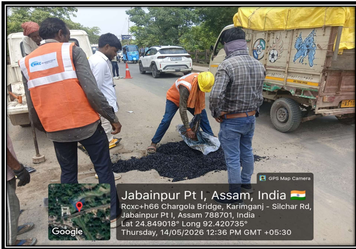
Port hole filling work in progress
