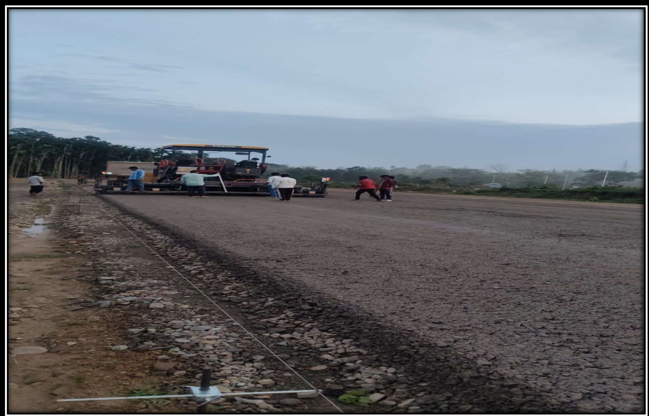
WMM Laying at CH-91+210 to 91+490 LHS
