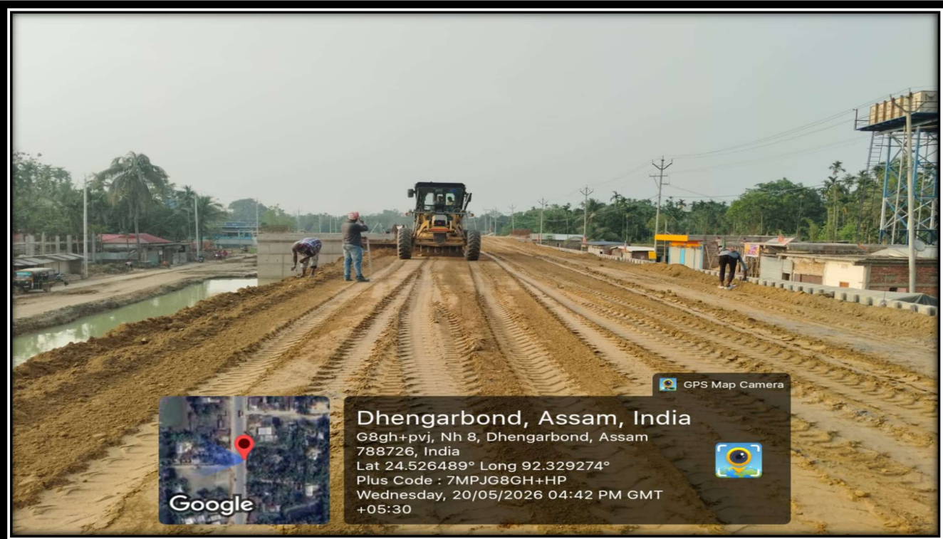
Subgrade Top Layer work in Progress at CH-92+260 to 92+360 LHS
