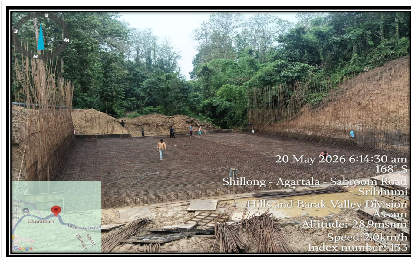
Reinforcement work in progress at CH-106+258 (MNB) Raft (BHS)
