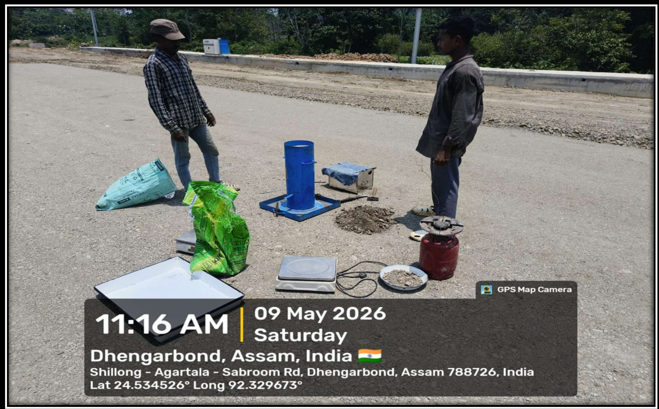
FDD Checking of WMM at CH-91+390 to 91+490 LHS
