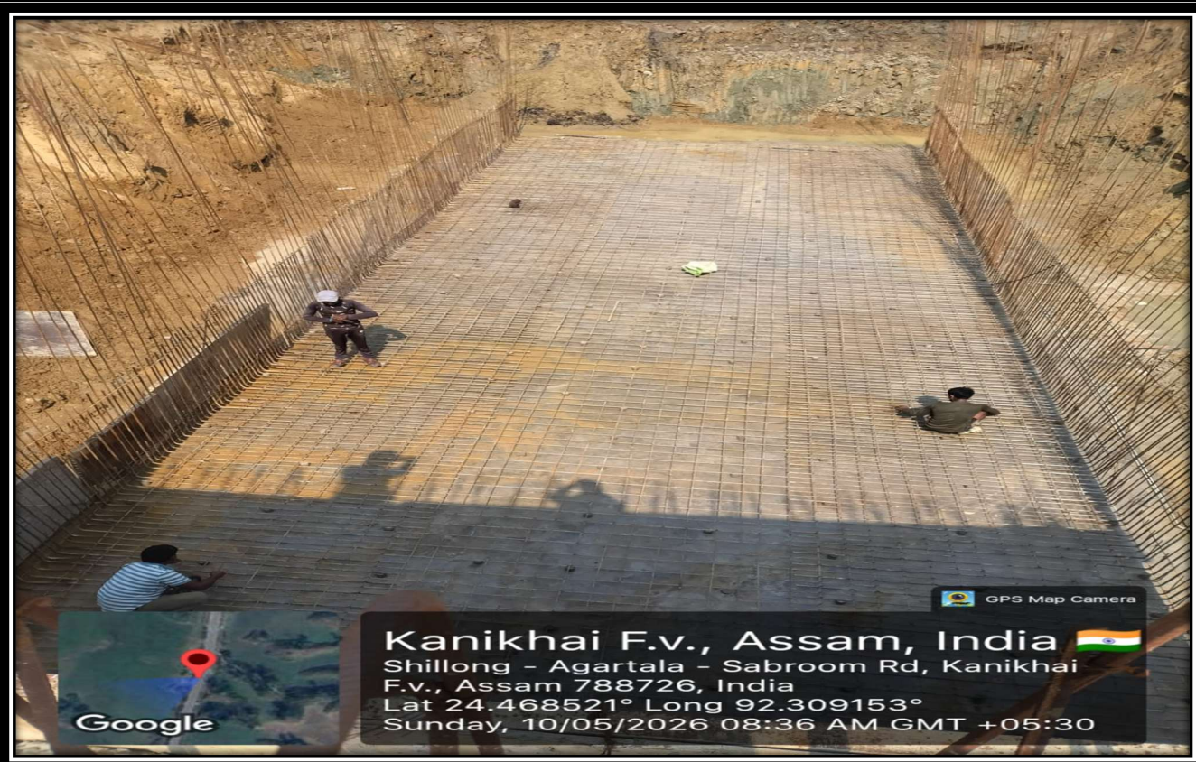
Reinforcement work in Progress at ch-99+250 RHS (MNB)
