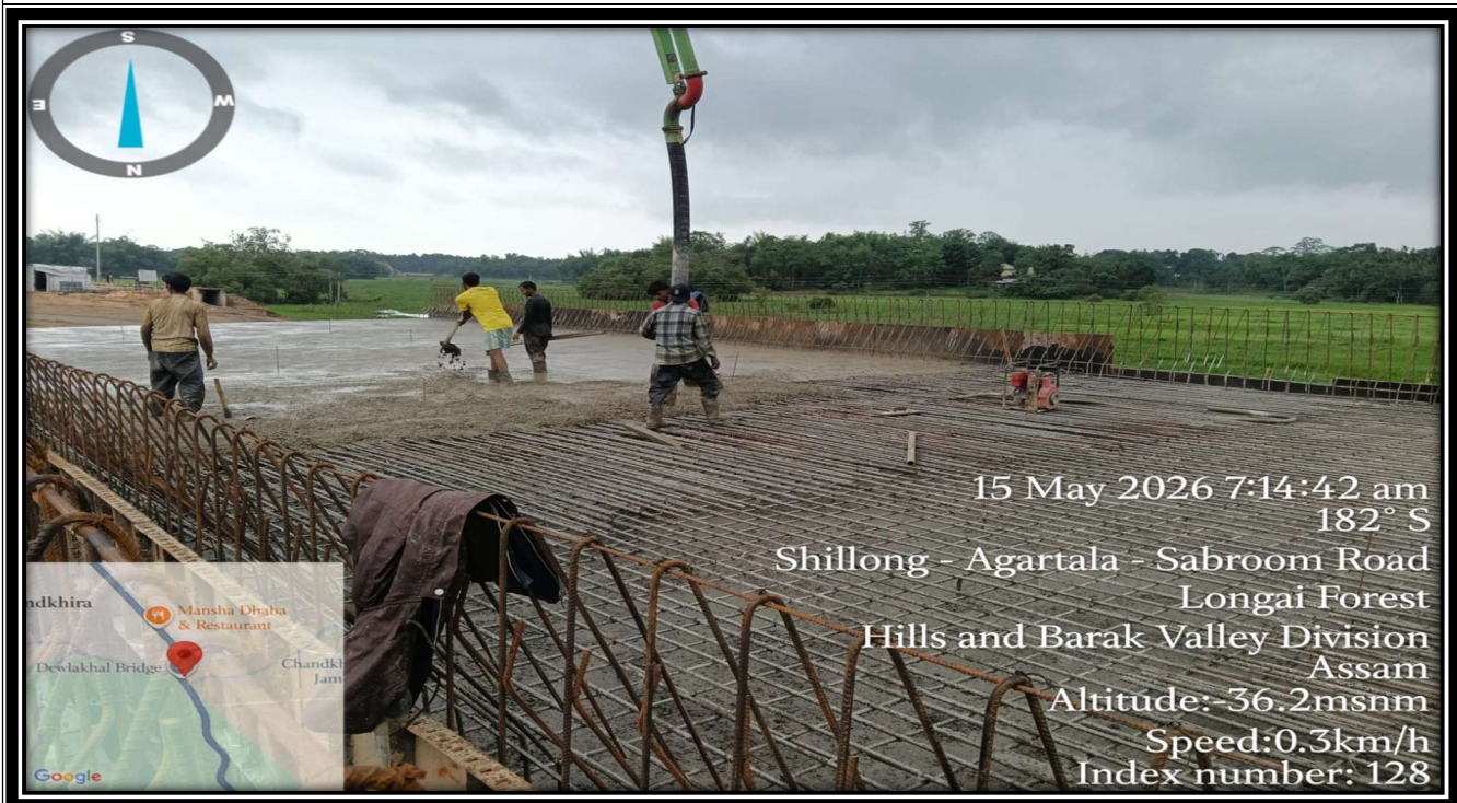
MNB Top Slab Concrete Pouring work in progress at CH-87+794 (RHS)
