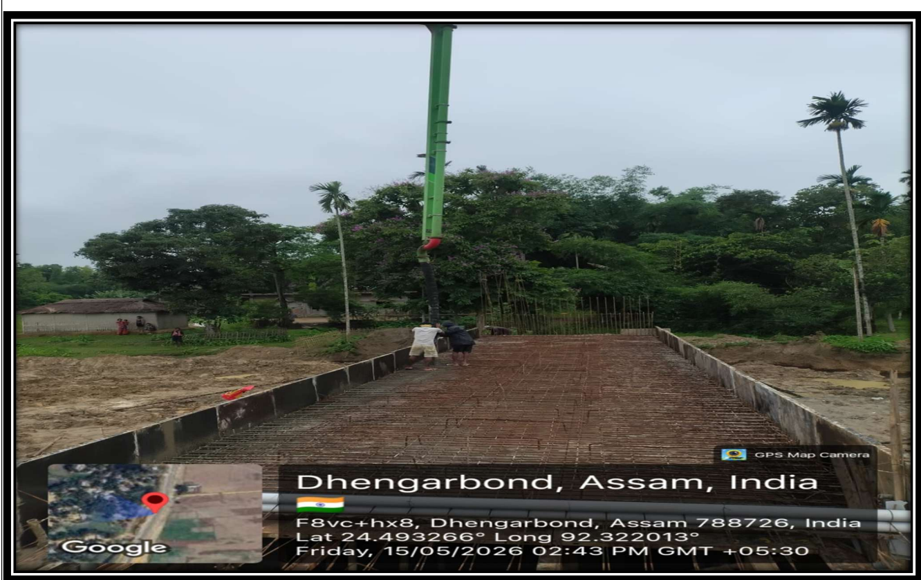
Box Culvert Top slab Concrete Pouring at CH-96+130 RHS
