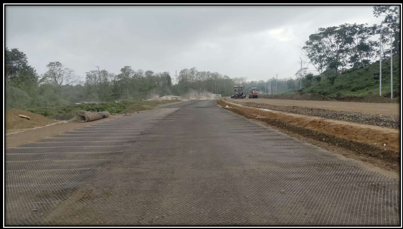
Geogrid Laying work in Progress at CH-101+430 to 101+610 LHS
