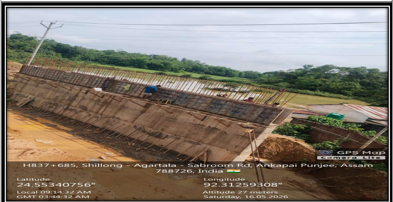
Retaining wall 4th lift stuttering fixing at CH- 88+540 to 88+560 LHS
