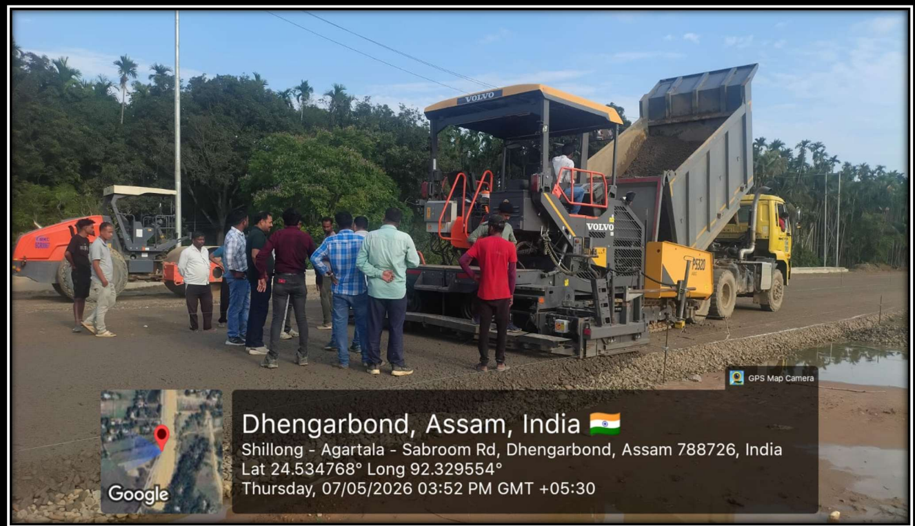
WMM Top Layer Laying at CH-91+210 to 91+490 LHS
