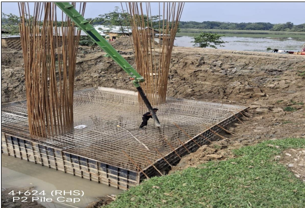
ROB P2(RHS)- Pile Cap Concrete Pouring
