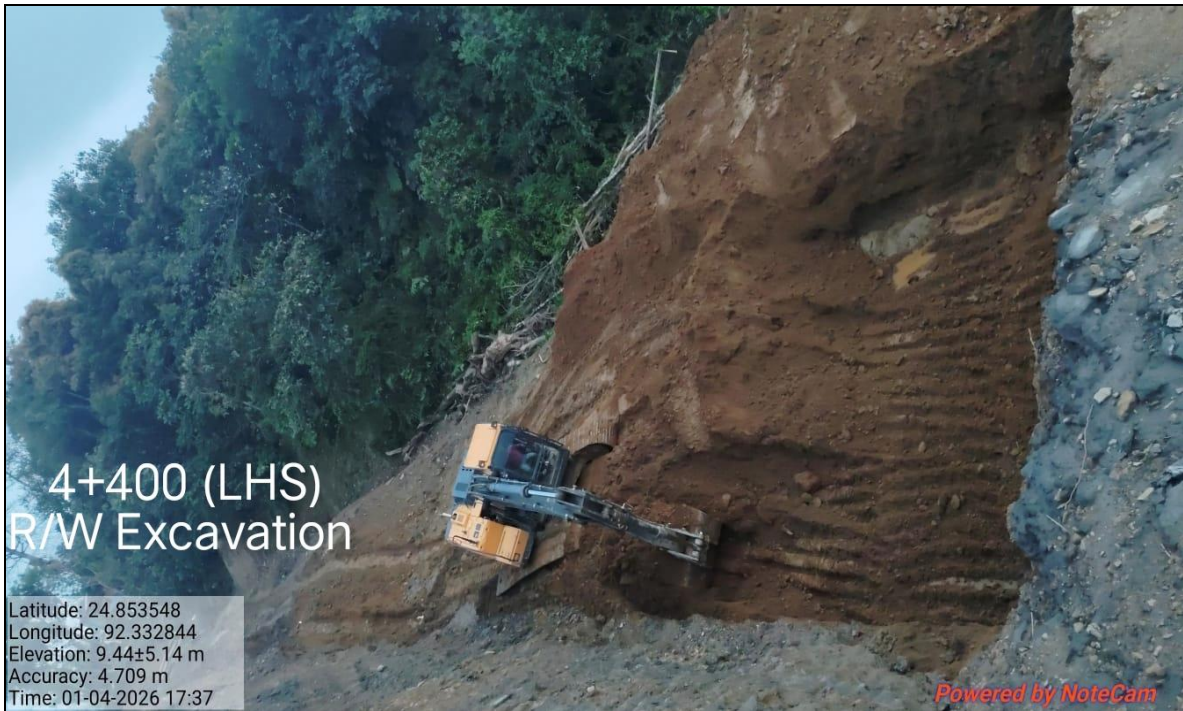
Retaining Wall Excavation Ch- 04+400
