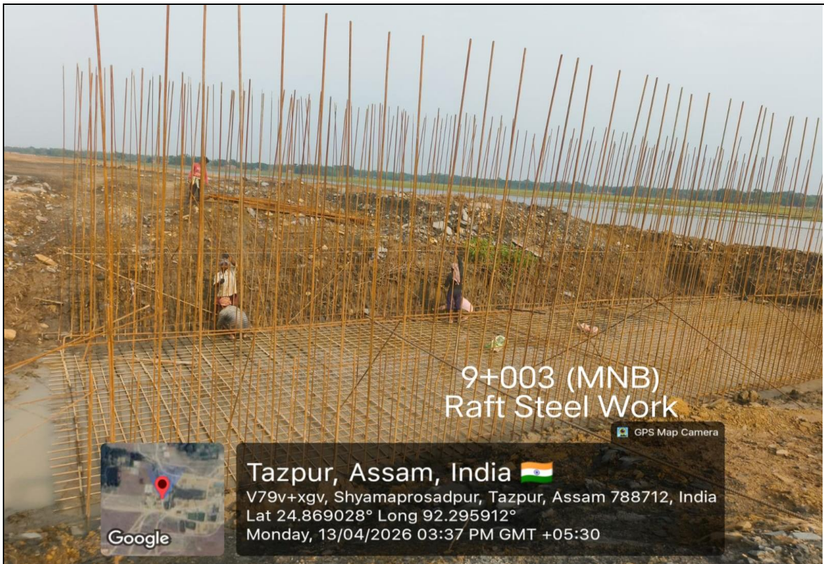
MNB- RAFT Steel Reinforcement Ch- 09+003
