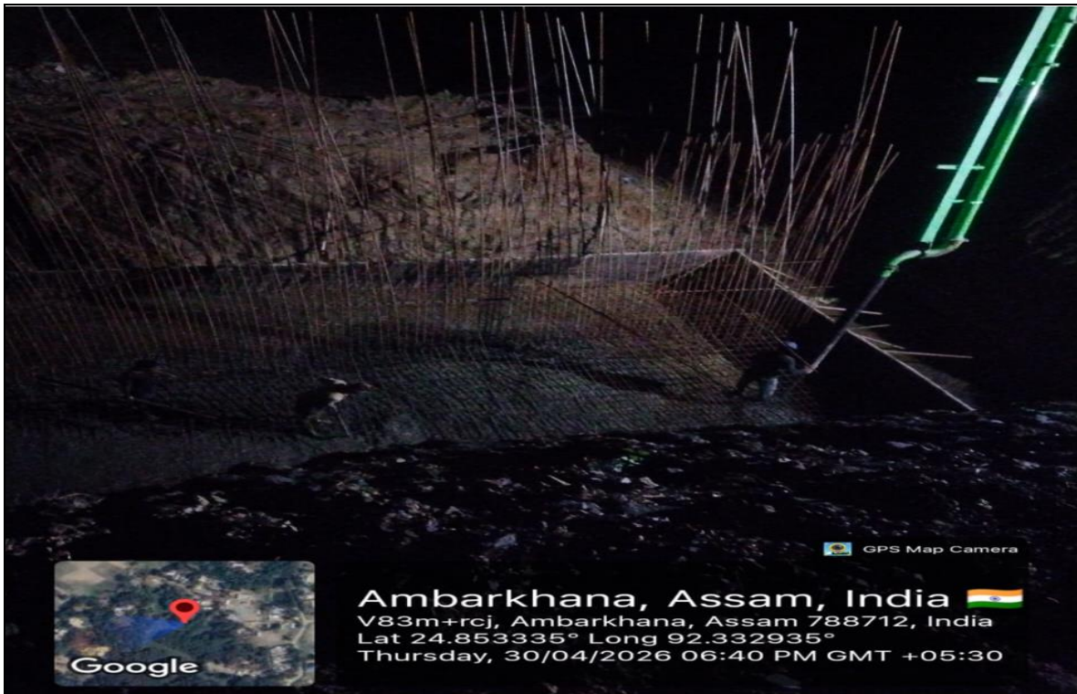
RETAINING WALL- RAFT Concrete Pouring Ch - 04+388
