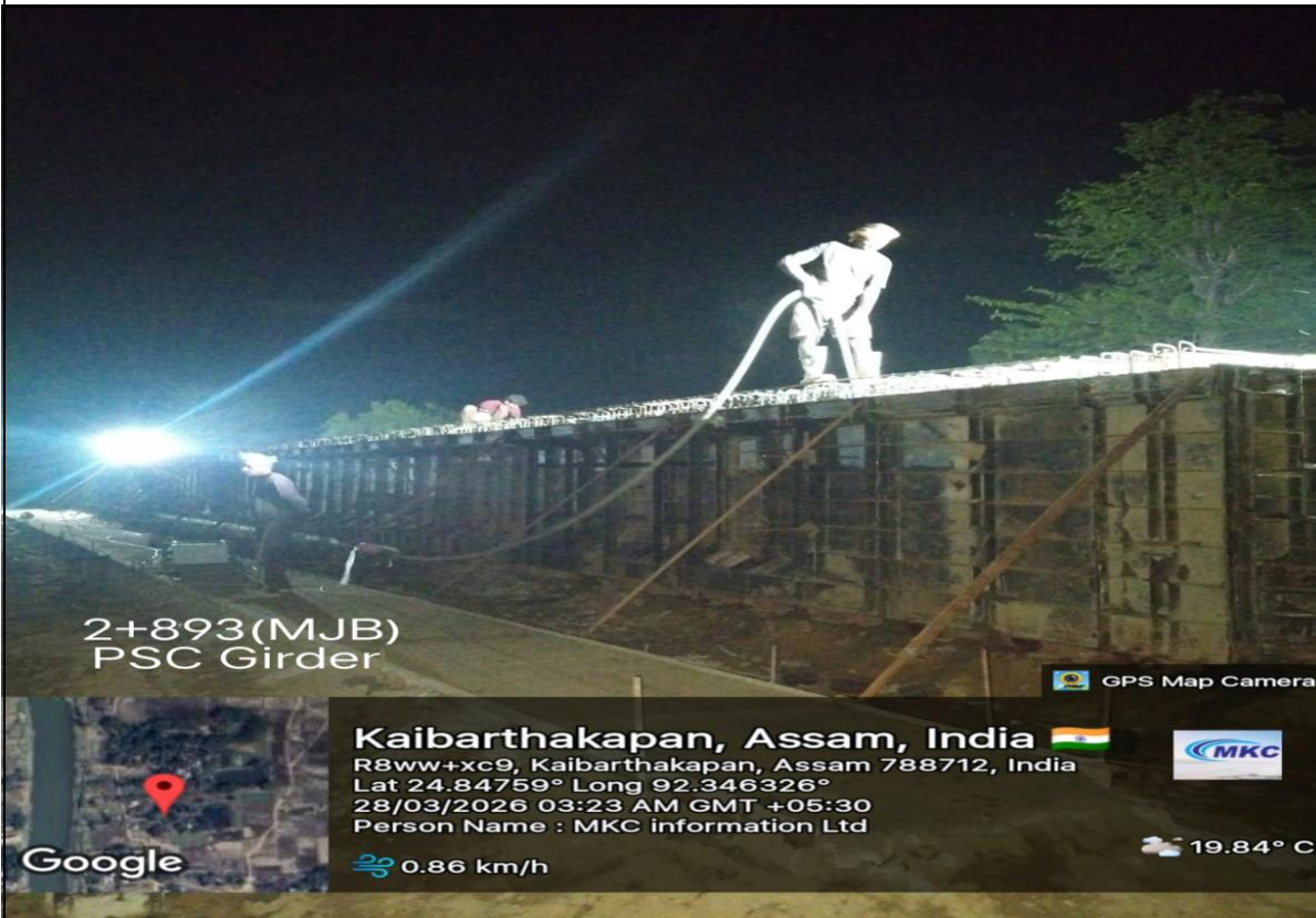
MJB- GIRDER Concrete Pouring Ch-02+893
