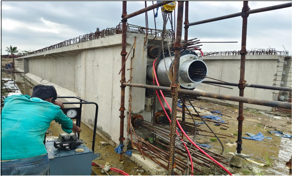
MJB PSC GIRDER-06 Stressing Ch- 00+526
