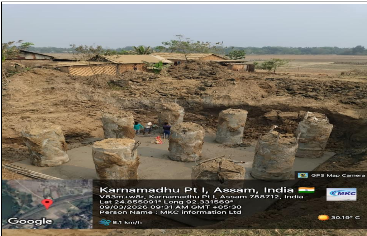
ROB- P2 PILE CHIPPING WORK AT CH-04+624
