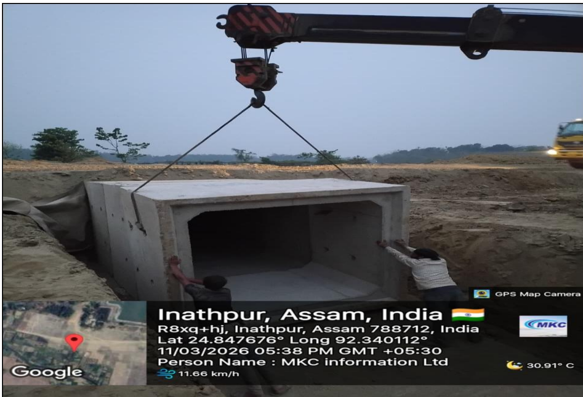
BOX CULVERT ERECTION IN PROGRESS At Ch- 03+418
