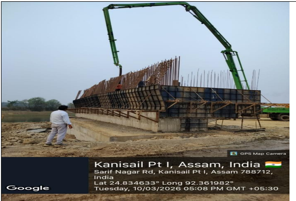
MJB- A1 ABUTMENT CAP CONCRETE POURING CH-00+526
