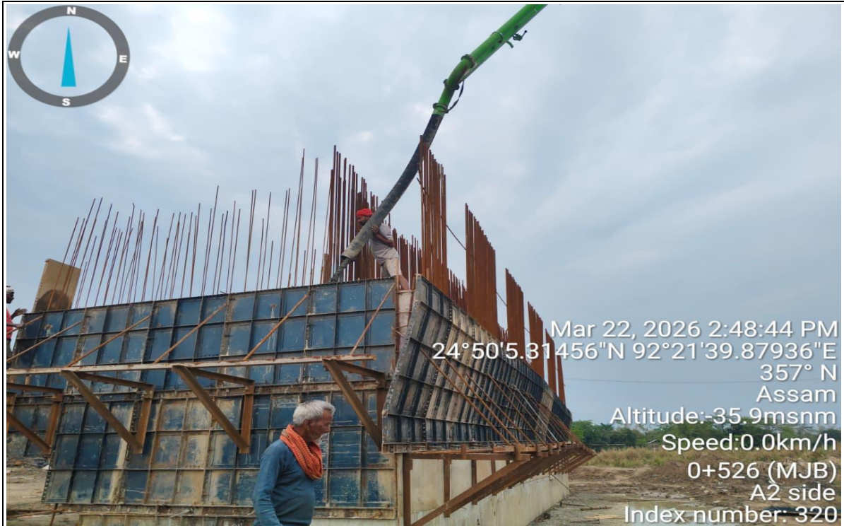
MJB- A2 ABUTMENT SHAFT FINAL LIFT CONCRETE POURING IN PROGRESS Ch-00+526
