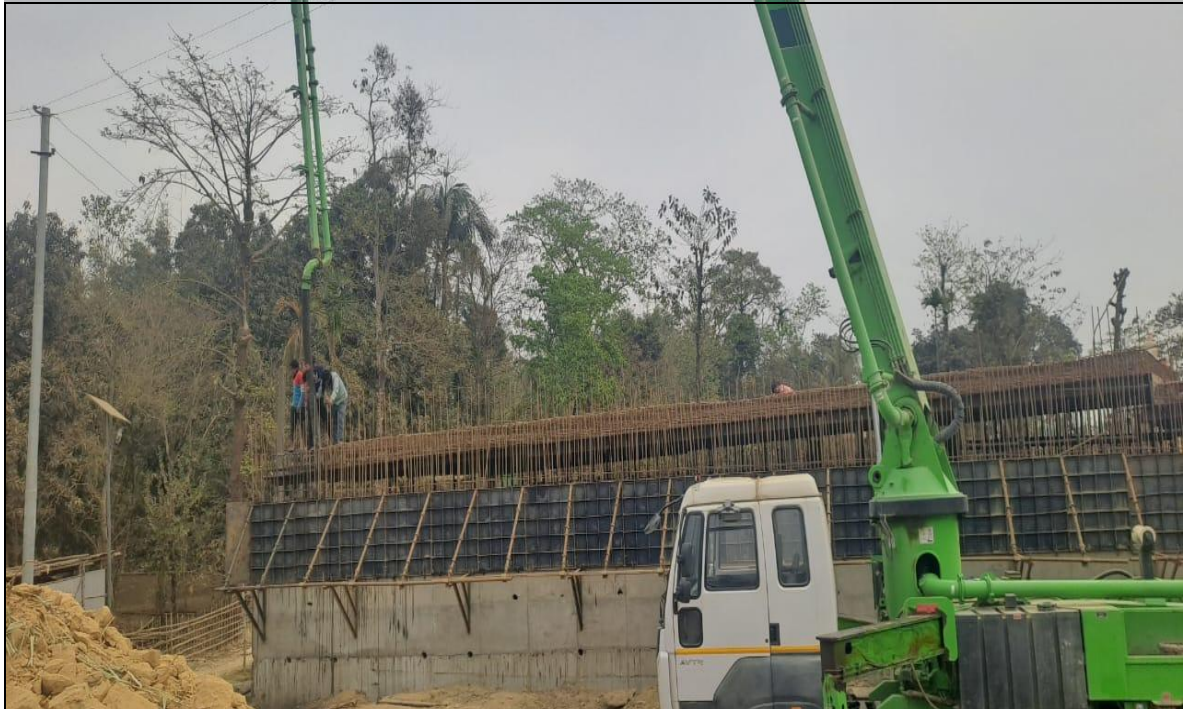
SVUP- 3 RD LIFT A1&A2 CONCRETE POURING IN PROGRESS Ch- 03+728
