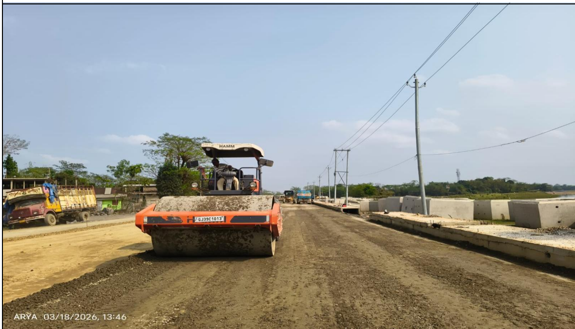
DLC TOP ROLLING WORK IN PROGRESS Ch- 13+200 To 13+260
