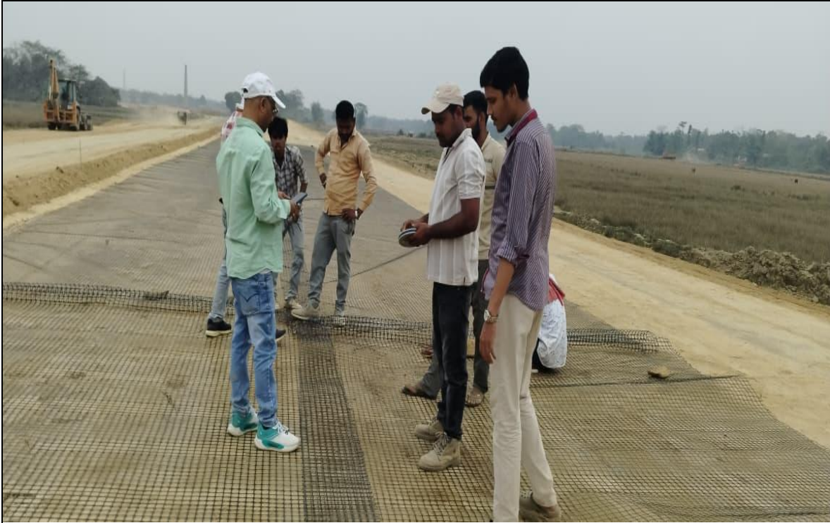
CLIENT INSPECTION FOR GEOGRID FIXING GSB LAYING 2+000 TO 2+100 LHS
