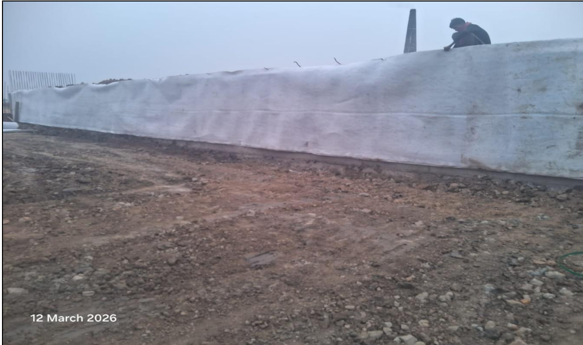
GEOCOMPOSITE FIXING CH- 00+213 At BOX CULVERT
