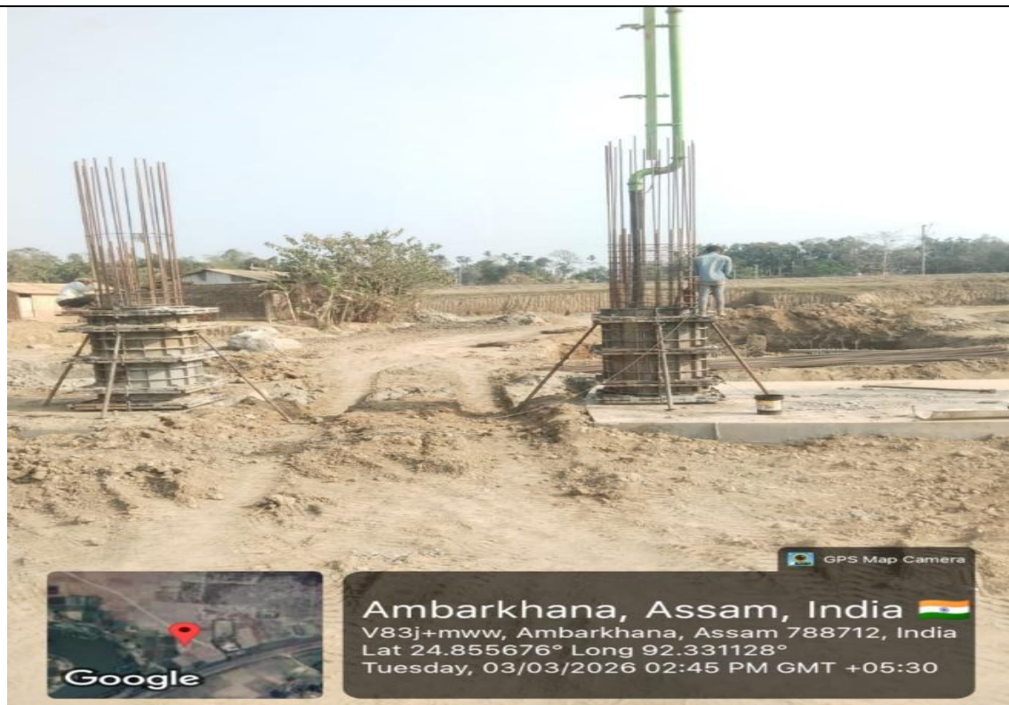
MJB- A2 ABUTMENT SHAFT FINAL LIFT CONCRETE POURING IN PROGRESS Ch-00+526
