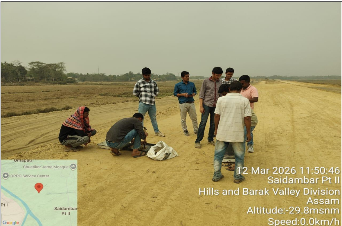
FDD TESTING FOR SUB-GRADE TOP LAYER CH- 01+800 TO 01+960
