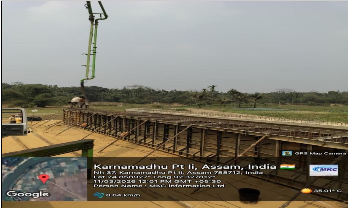
GIRDER CONCRETE POURING CH-05+332 At MJB
