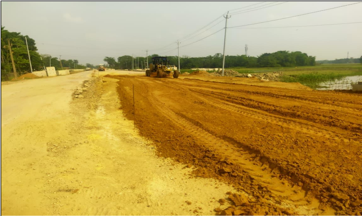
SG Top Preparation at Ch- 13+040 to 13+110 LHS
