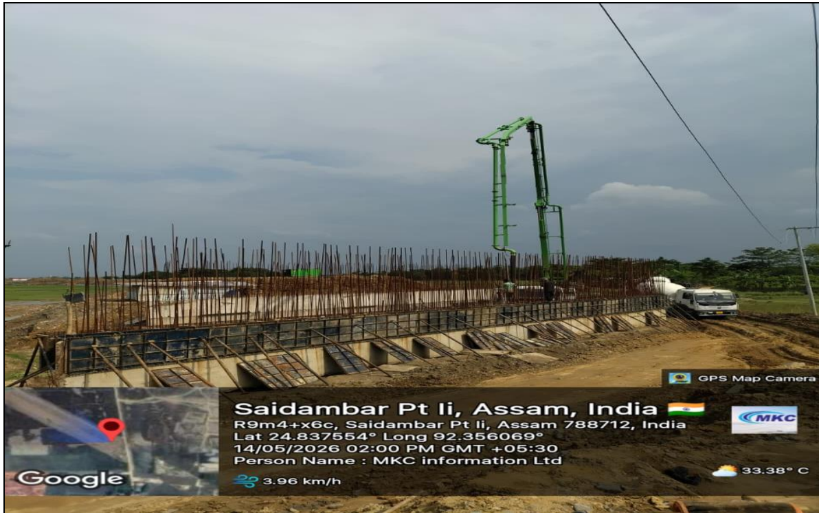
LVUP- A2 2 nd Lift Concrete Work at Ch- 01+142
