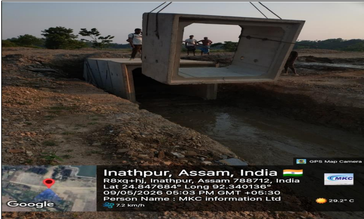
Box Culvert Erection Work at Ch- 03+418
