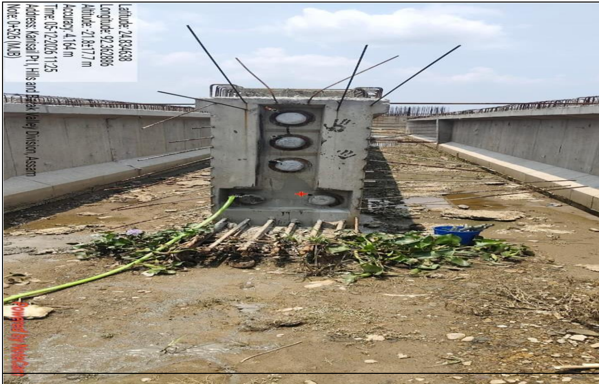
MJB- PSC GIRDER GROUTING( G-04) at Ch- 00+526
