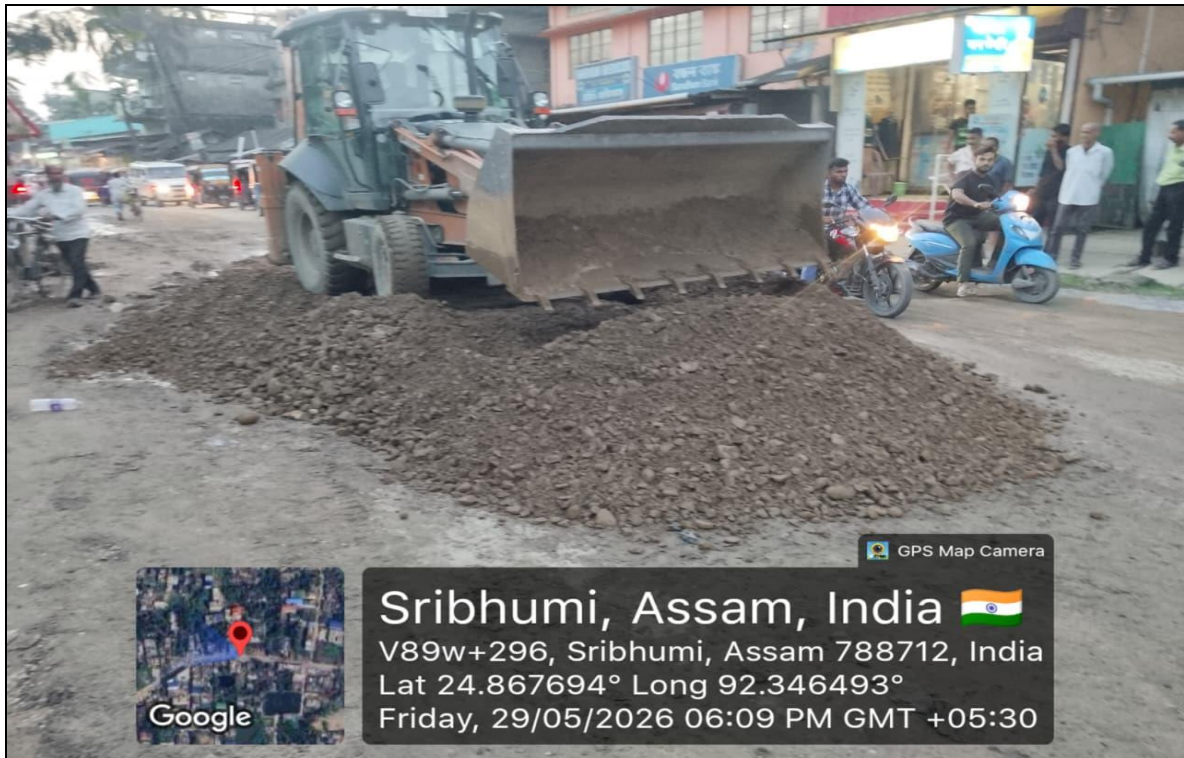
GSB filling for pot hole at settlement
