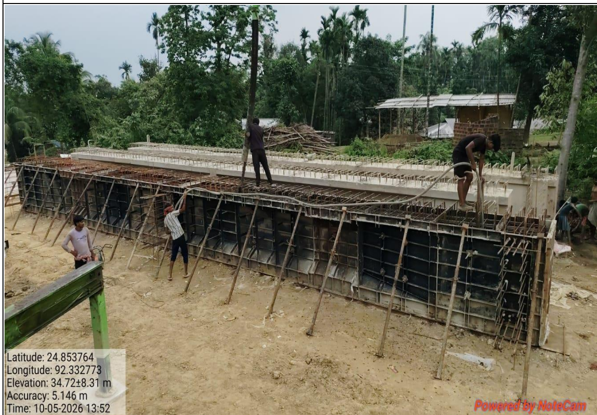
ROB- G-03 GIRDER Concrete Work at Ch- 04+624
