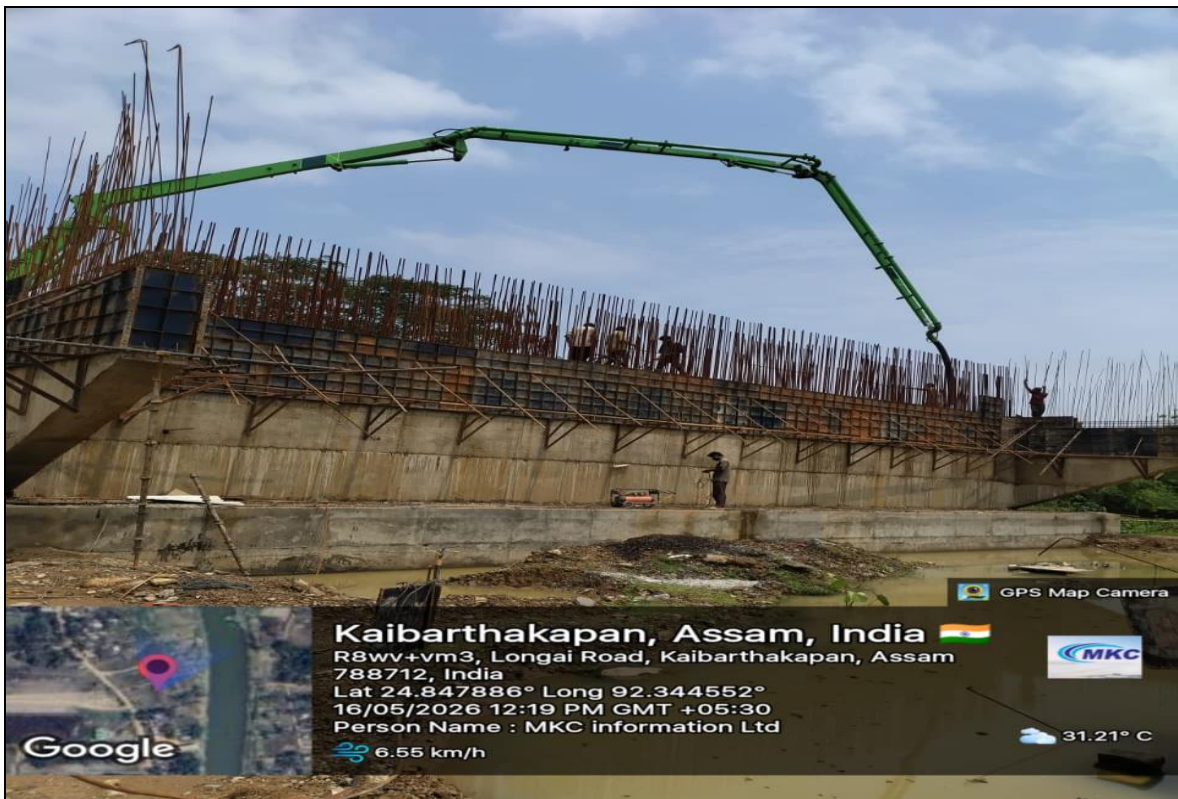
MJB- A2 ABUTMENT CAP Concrete Work at Ch- 02+893
