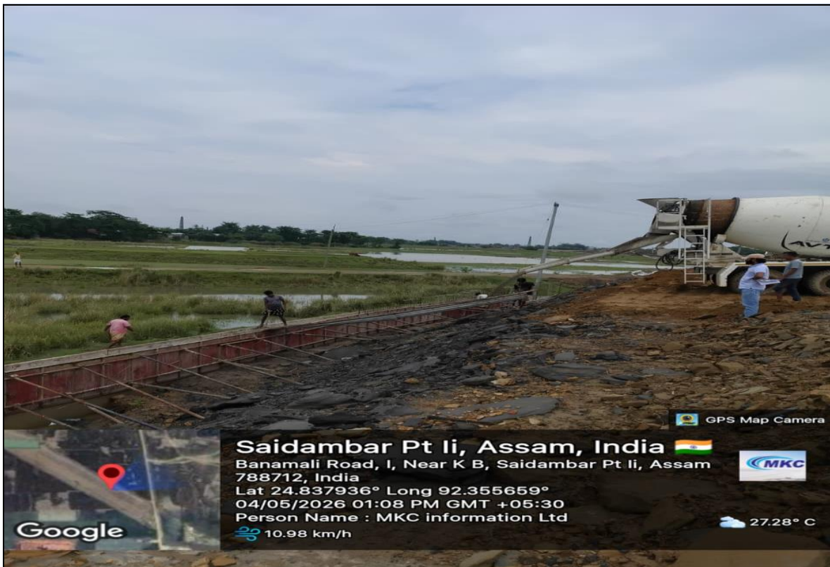
TOE WALL Final Lift Concrete Work at Ch- 01+203 to 01+227 RHS
