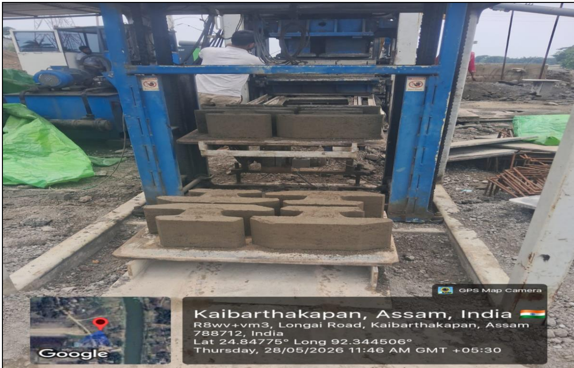
RE Block casting work
