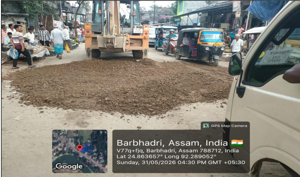
Fakira bazaar main market road maintenance work
